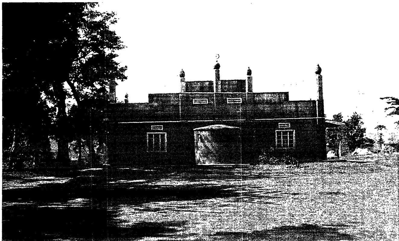
Fig. 2. Kampala, Uganda. The modern Kasubi mosque.
