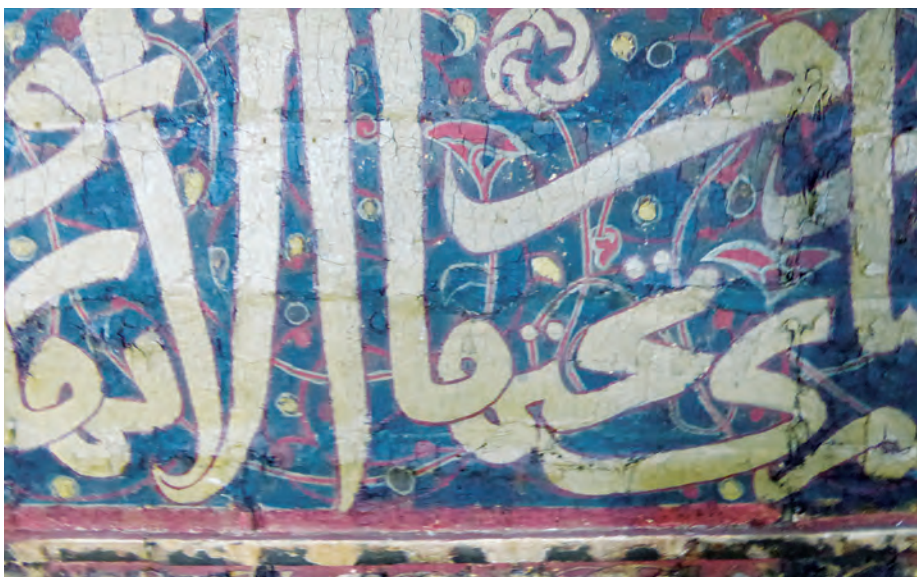
Above: Injections of adhesive to reattach peeling paint complement the use of a hot spatula to return the detached flakes to their original position (AKTC Conservation Team, 2020).
