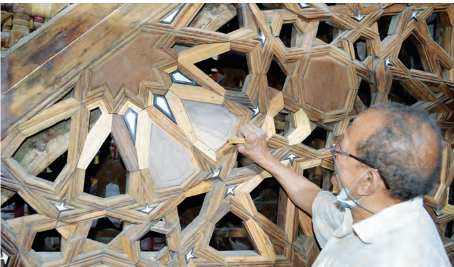
Above: Manufacturing the individual inlaid pieces to be mounted on the panels (AKTC Conservation Team, 2020).
