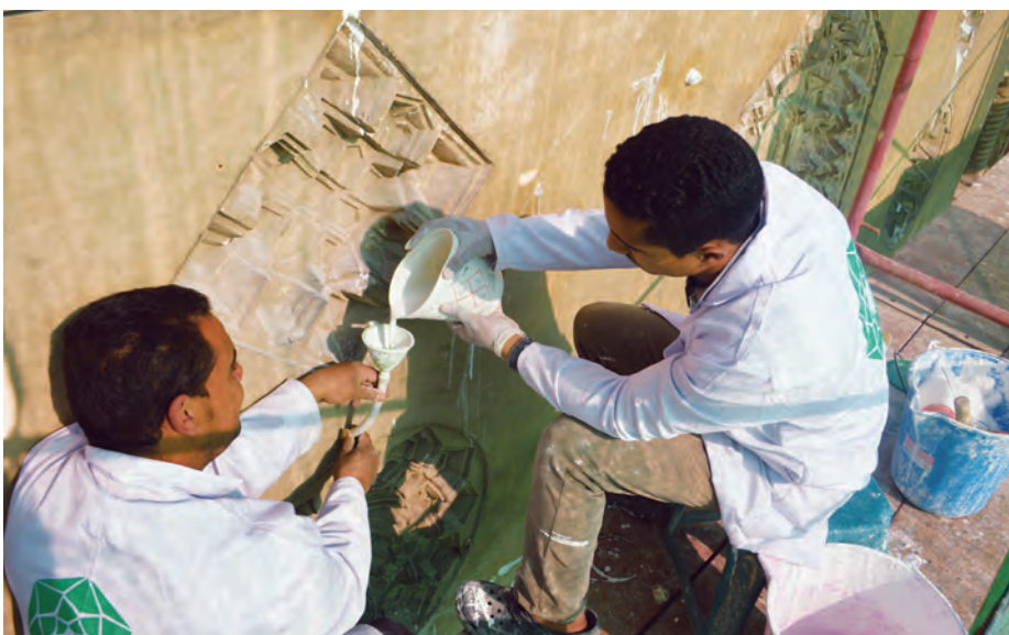
Above: Cleaning by hand the ornamental plaster muqarnas in one of the finials located at the corner of the mosque (AKTC Conservation Team, 2021).
