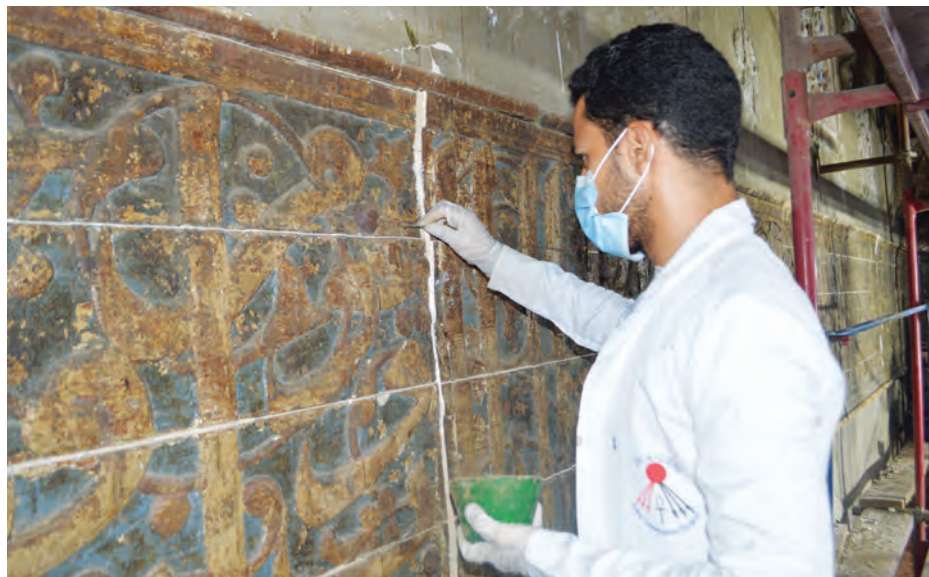
Below: Filling the minor gaps between timber planks with wood dust mixed with acrylic resin with adhesive properties (AKTC Conservation Team, 2020).
