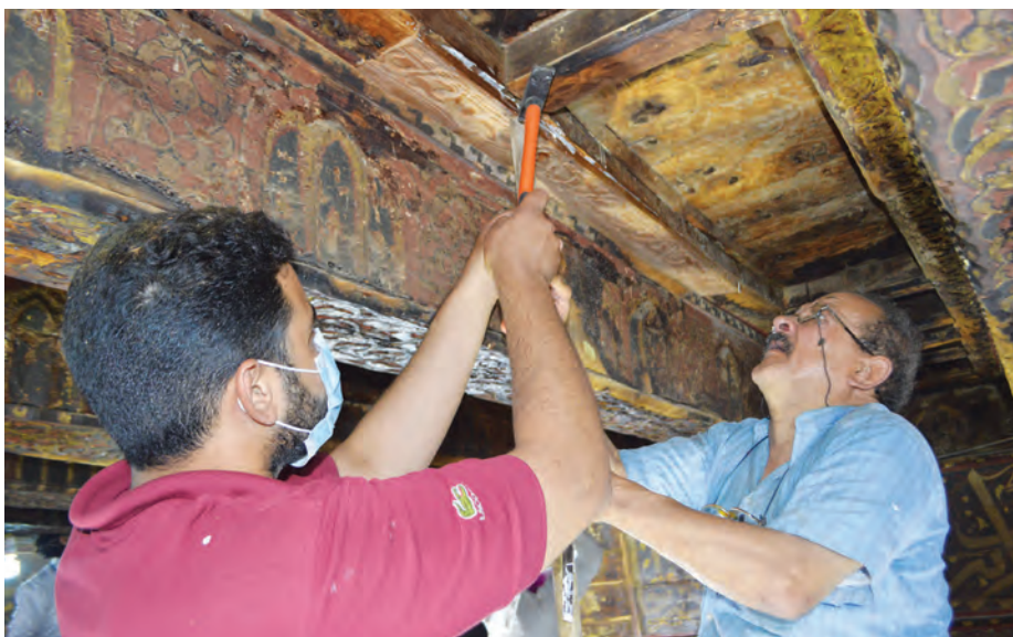
Above: Manual cleaning with the use of a small scalpel to remove black crust (AKTC Conservation Team, 2020).
