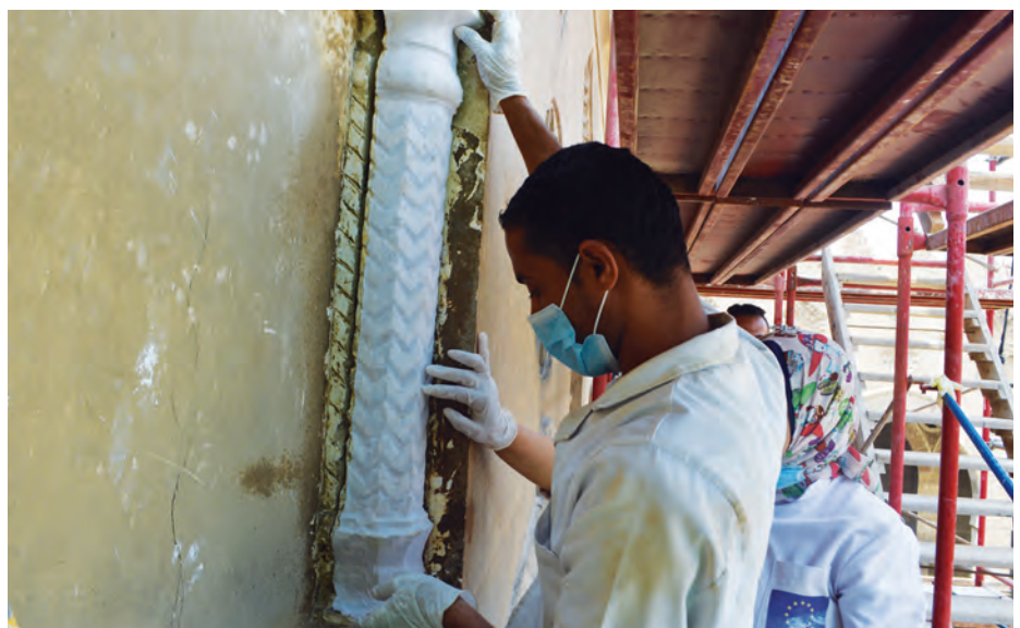
Middle: Re-attaching the bulb finial on top of a crenelation (AKTC Conservation Team, 2021).
