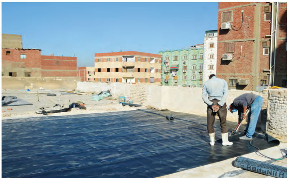
Below: Installation of the waterproof membrane made of torch-applied bitumen sheets (AKTC Conservation Team, 2020).
