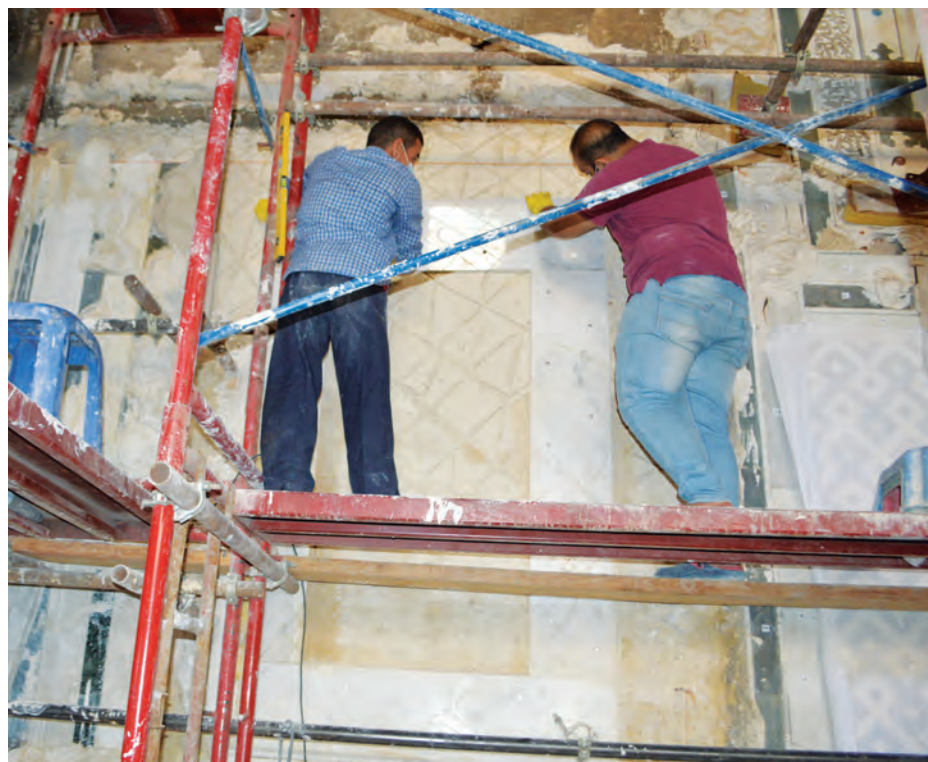
Below: Positioning of plain marble slabs on the qibla wall to serve as insulation and support for the subsequent re-instatement of the polychrome marble panels and mosaic decoration (AKTC Conservation Team, 2020).
