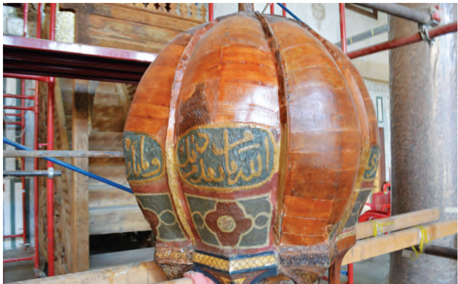
Middle: Shellac finish applied to the ebony and bone inlaid elements of the minbar (AKTC Conservation Team, 2020).
