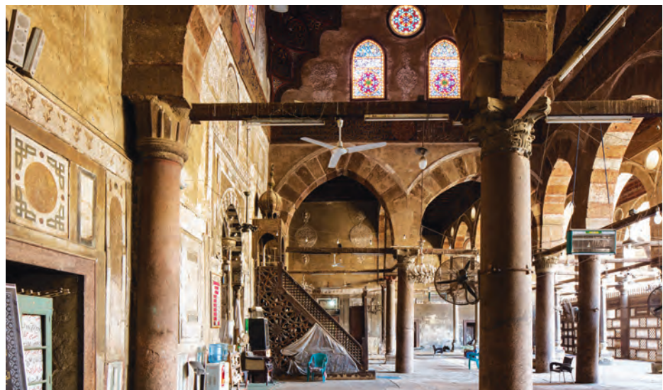
Right: View of the prayer hall looking south before restoration (Christian Richters, 2017).
