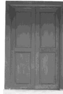
Figure 17. The detail of the window
