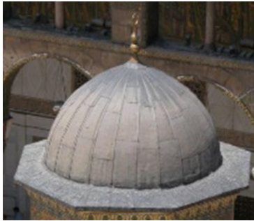
Figure 18: The octagonal cornice topped with a covering dome with plates of lead in the Umayyad Mosque in Damascus [29]
