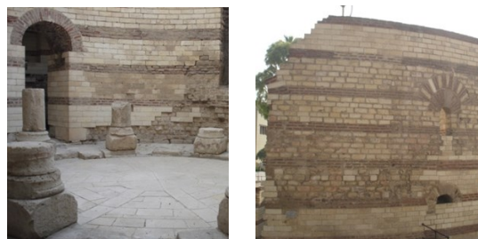
Figure 17: General view of the exchange of the stone courses and brick courses in the walls of the Babylon Fortress in Cairo (Author)
