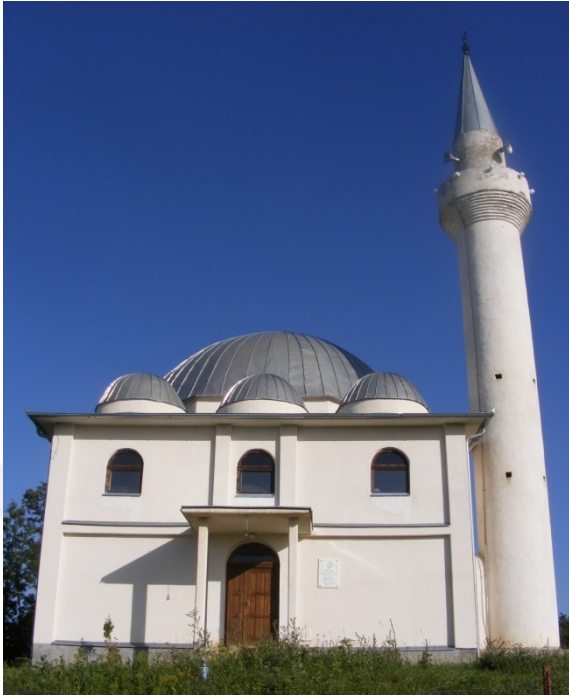
Fig. 1.1 Main / front, north-west facade
