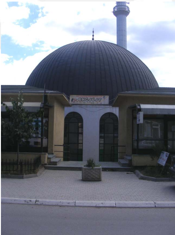
Fig. 1.7 Side facade, north-east
