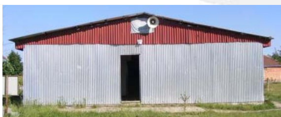
Fig. 1.1 Front/main facade, north-west
