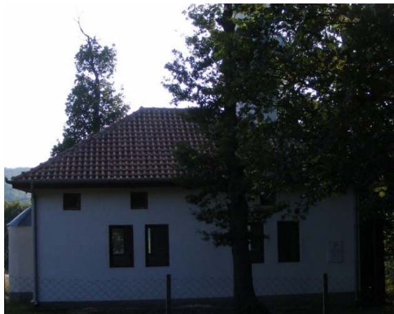
Fig. 1.7 Side facade, north-east
