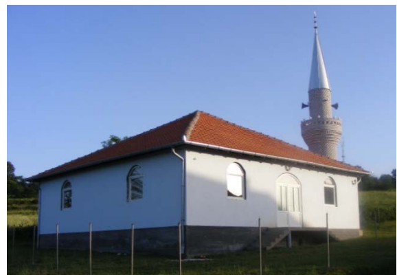
Fig. 1.7 View from north
