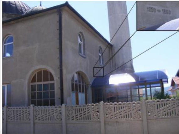
Fig. 2.2 View from north-east
