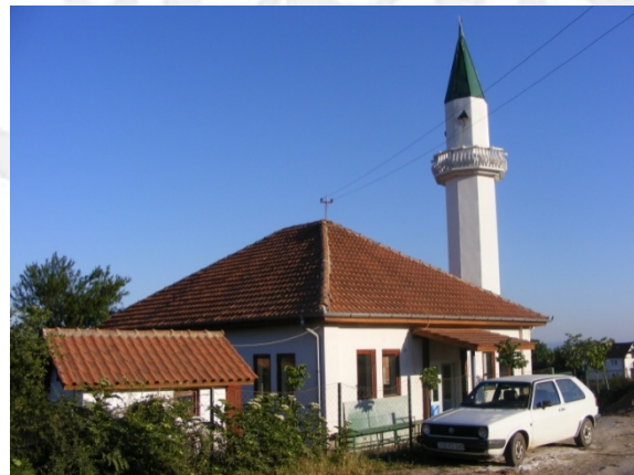
Fig. 1.8 View from north
