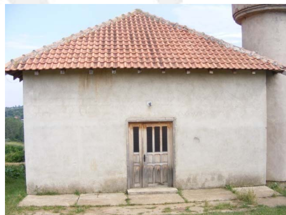
Fig. 1.1 Main / front, north-west facade
