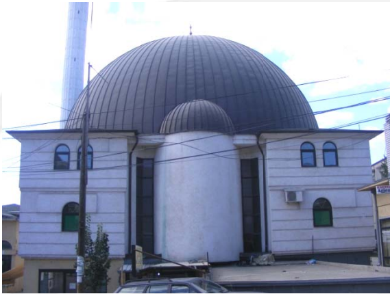
Fig. 1.5 Back façade, southeast
