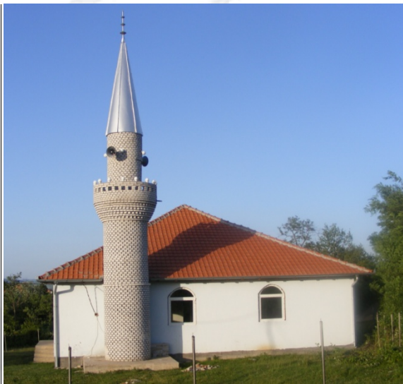
Fig. 1.3 Side facade, south-west
