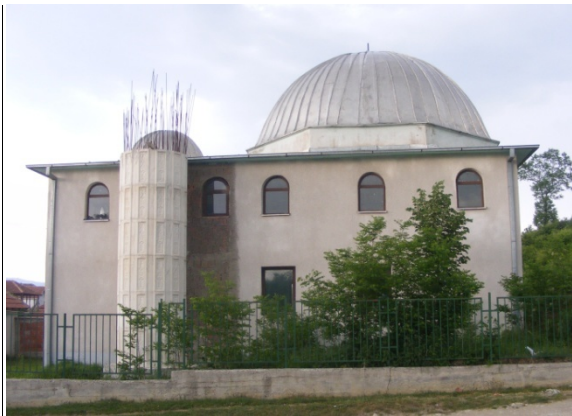
Fig. 1.3 Side facade, south-west
