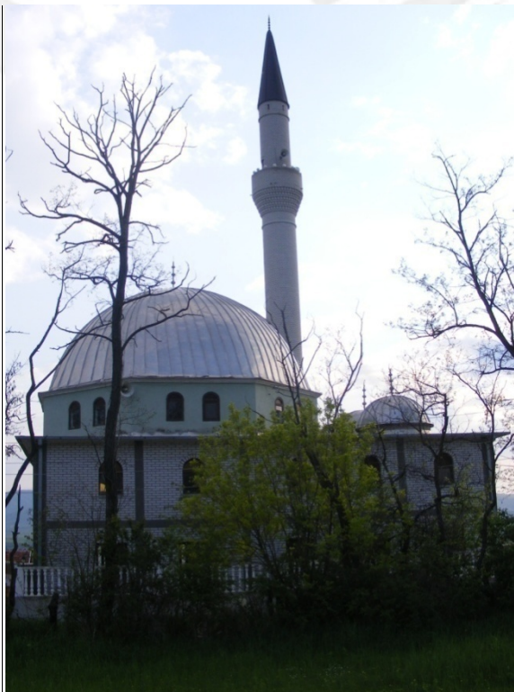
Fig. 1.7 Side facade, north-east
