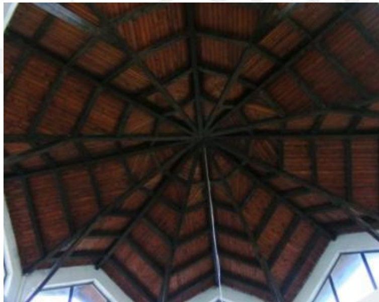
Fig. 4.4 Interior view of the 16-shed roof
