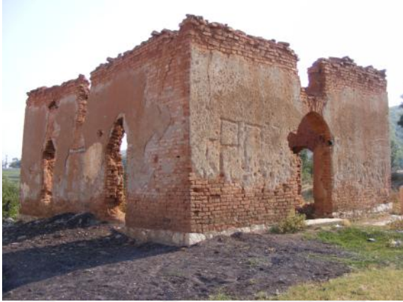
Fig. 1.7 View from north-east
