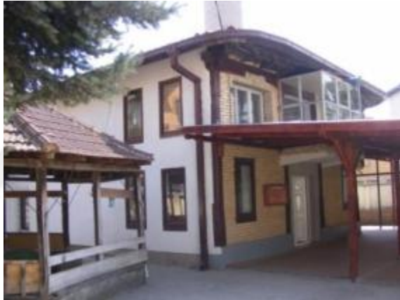
Fig. 1.4 View from North-east – the later Annex
