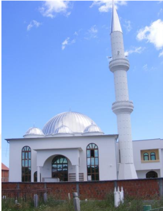
Fig. 1.1 Front/main facade, north-west
