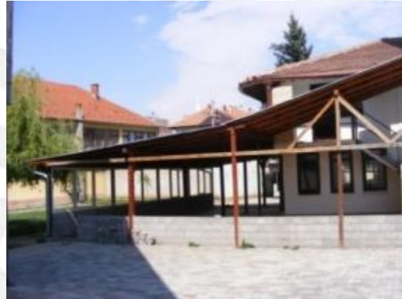
Fig. 1.5 View from south-west-façade – the new Annex (1999)
