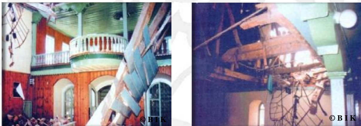
Fig. 2.3 and fig. 2.4 Interior view, after the war (1999)
