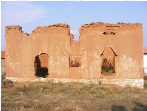
Fig. 1.3 Side facade, south-west
