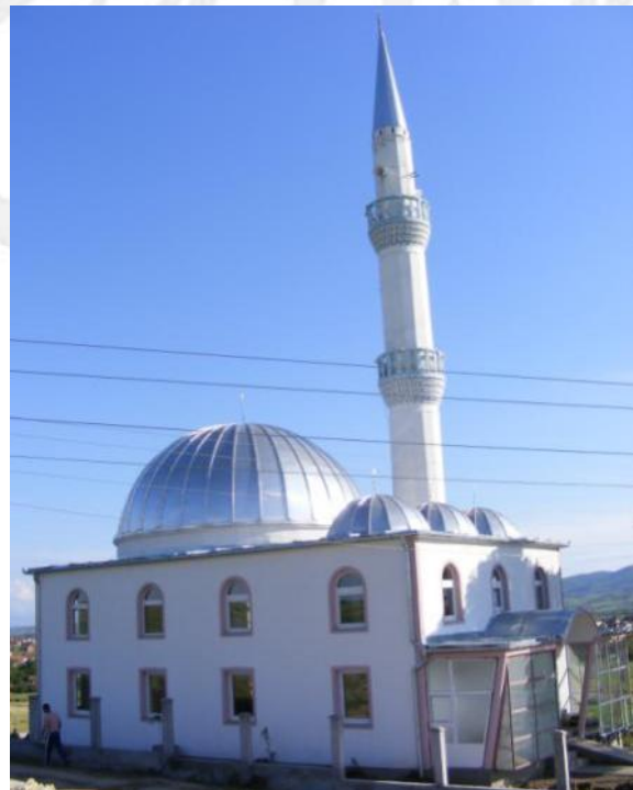
Fig. 1.8 Side facade, north
