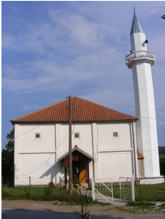
Fig. 1.1 Main / front, north-west facade
