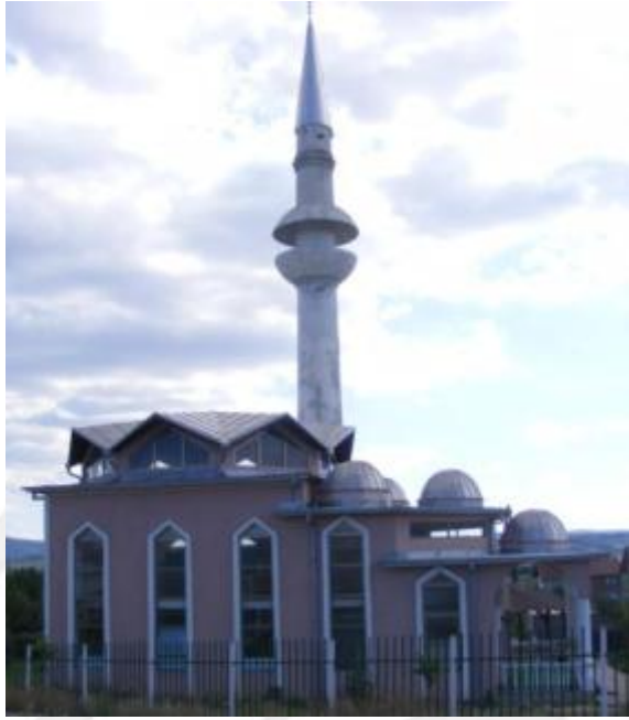
Fig. 1.5 View from northeast
