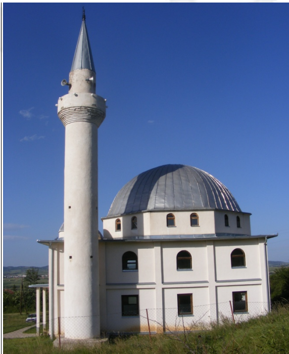
Fig. 1.3 Side facade, south-west
