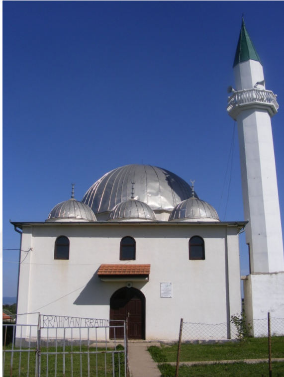
Fig. 1.1 Main / front, north-west facade
