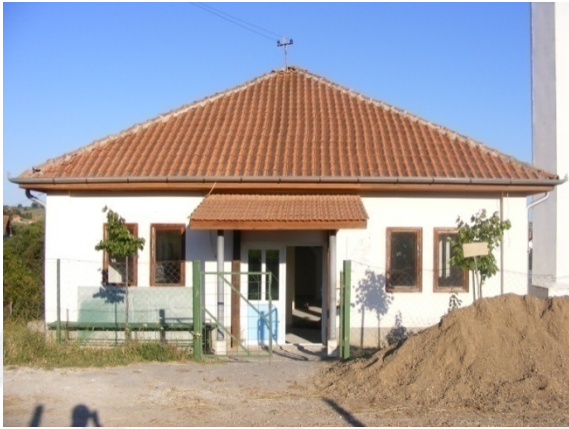
Fig. 1.1 Main / front, north-west facade
