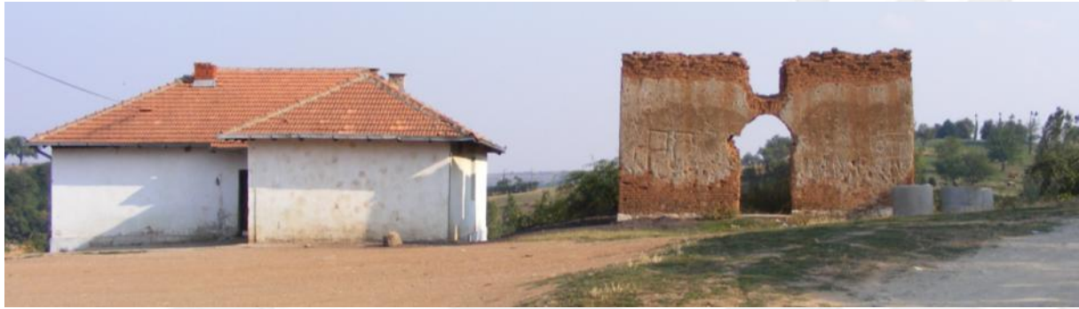
Fig. 4.1 View from the north-west, the school on the left and the mosque on the right
