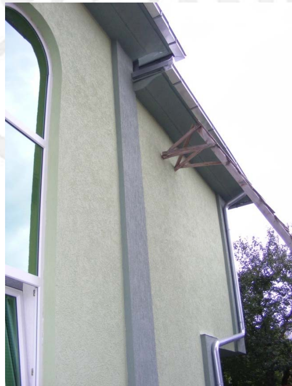
Fig. 1.8 Side facade, north-east
