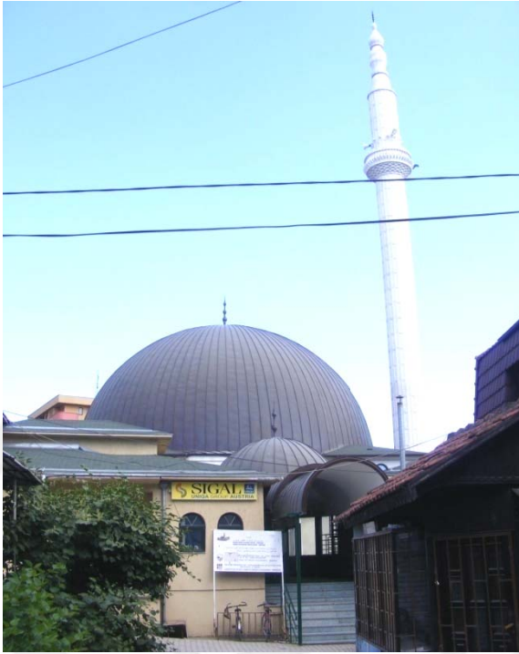
Fig. 1.1 Main / front, north-west facade
