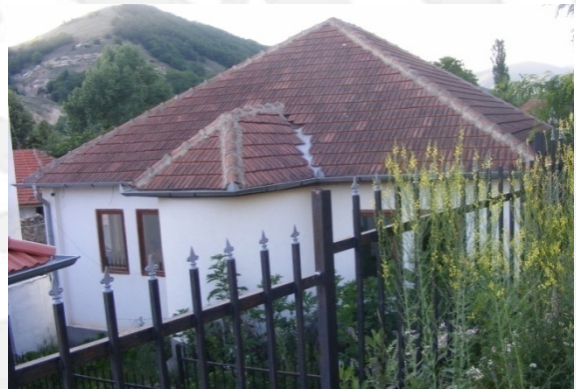
Fig. 1.4 Back facade, south
