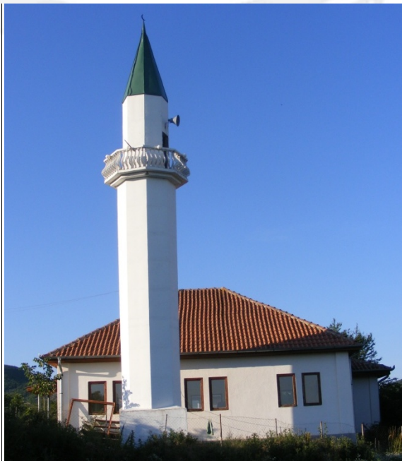
Fig. 1.3 Side facade, south-west
