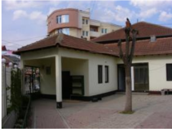
Fig. 2.1 View from north 9
