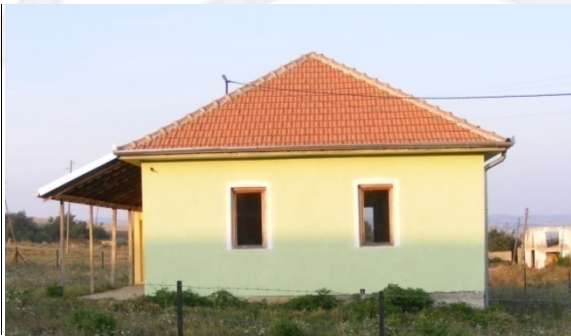
Fig. 1.3 Side facade, south-west
