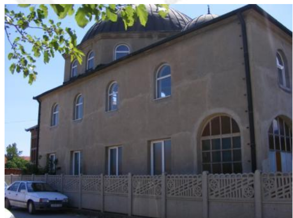
Fig. 1.4 Side facade, north-east
