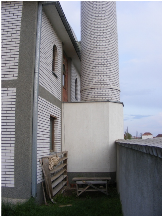
Fig. 8.2 View from the ground of the minaret
