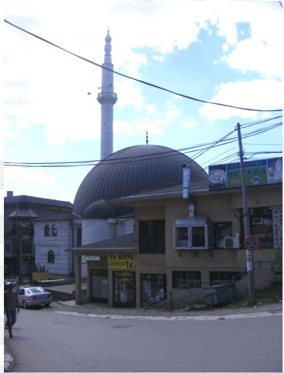
Fig. 1.6 View from north-east
