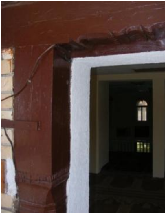
Fig. 1.25 Interior detail – upper floor, the bolster and the pile.
