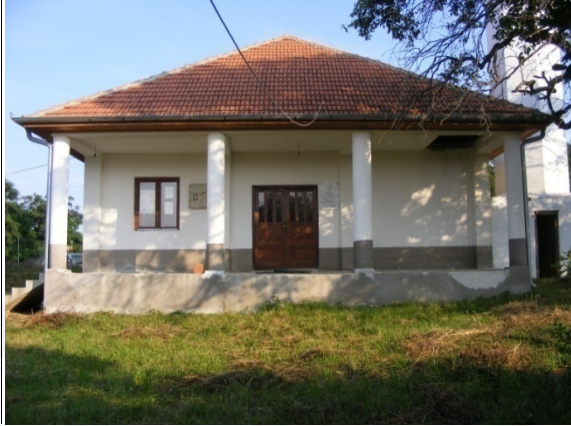
Fig. 1.1 Main / front, north-west facade
