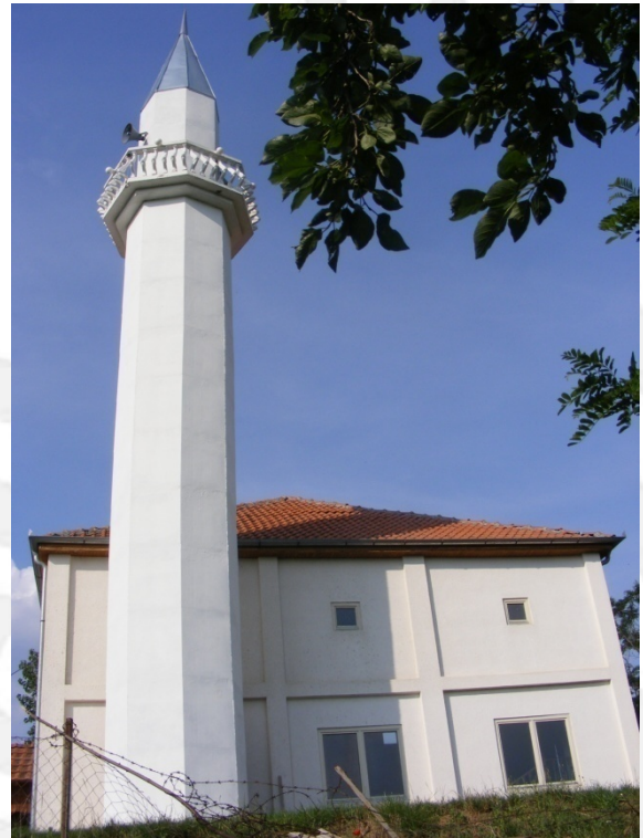
Fig. 1.2 Side facade, south-west
