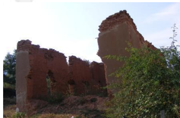
Fig. 1.6 View from south-east
