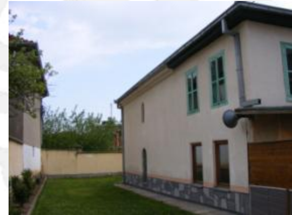
Fig. 2.4 View from south-east
