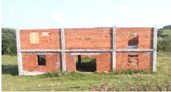
Fig. 1.1 Main / front, north-west facade
