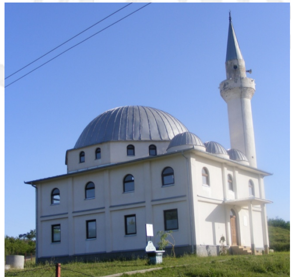
Fig. 1.8 View from north
