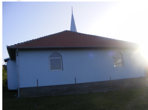
Fig. 1.6 Side facade, north-east
