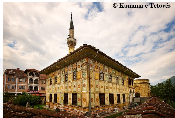
Fig. 5.14 Spotted Mosque in Tetovë from east
