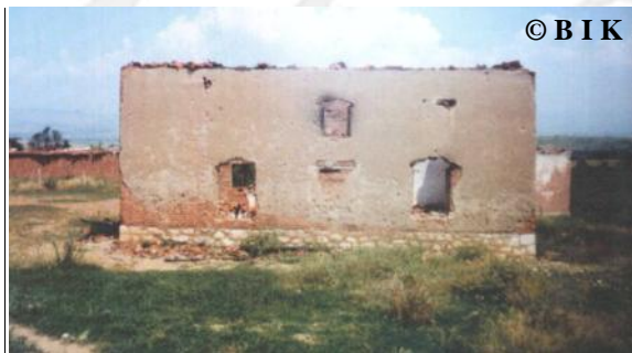
Fig. 4.2 An after war view (1999) from south-west
