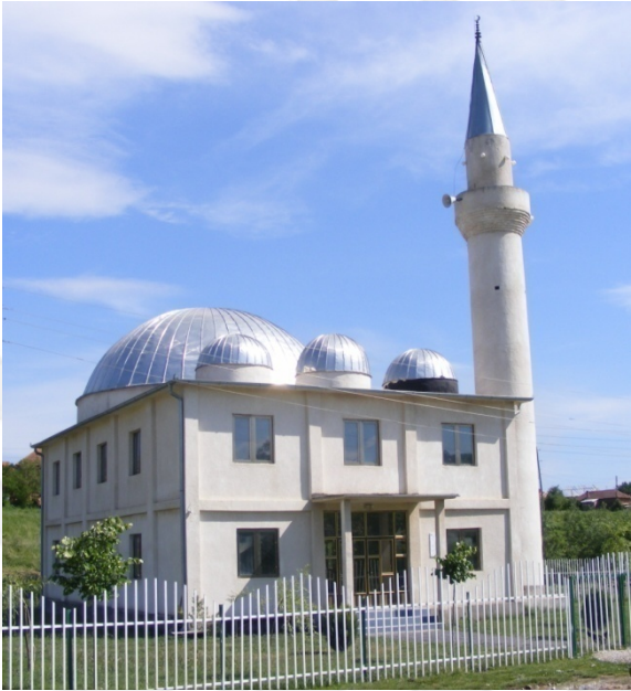
Fig. 1.8 Side facade, north
