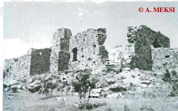
Fig. 5.12 Lezhë, Kala (Castle) Mosque, from south
