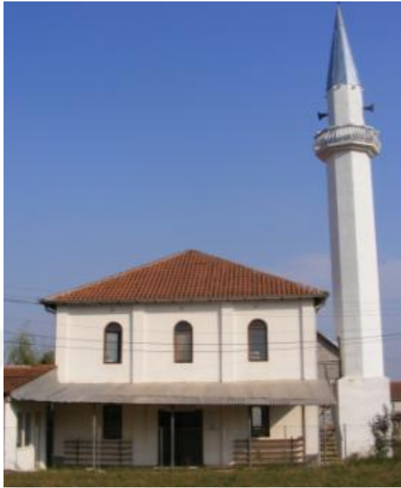
Fig. 1.1 Front/main facade, north-west
