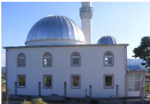
Fig. 1.7 Side facade, north-east
