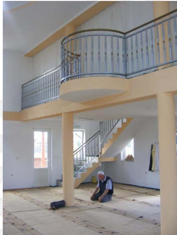
Fig. 7.4 The gallery/ upper floor; a view of the construction slab
