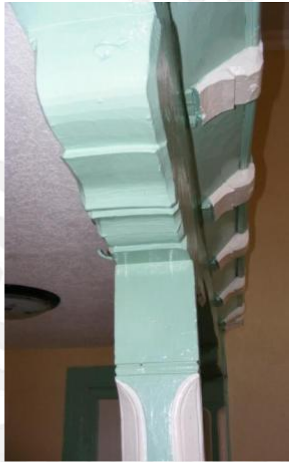
Fig. 1.23 Interior detail under the gallery slab: the top of the pillar with the typical bolster.
