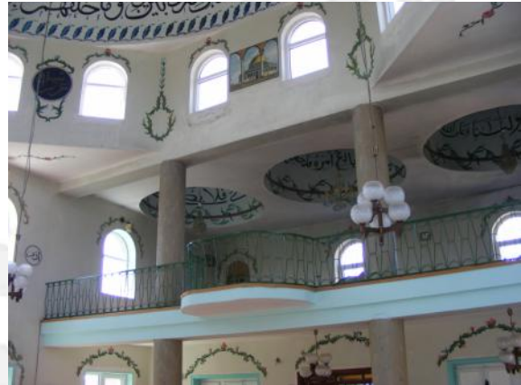
Fig. 2.3 The gallery floor/mafil, the armoured concrete slab
