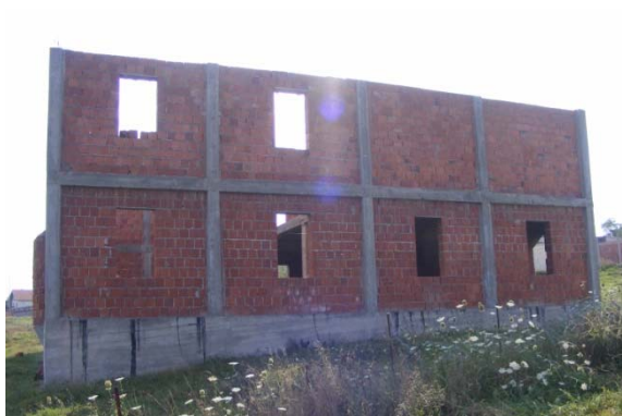
Fig. 1.7 Side facade, north-east
