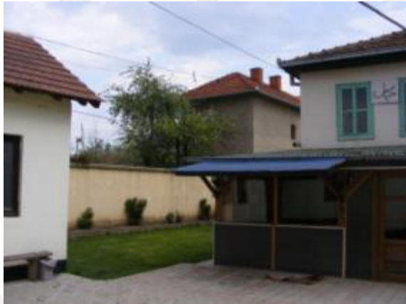
Fig. 2.3 View from south-east
