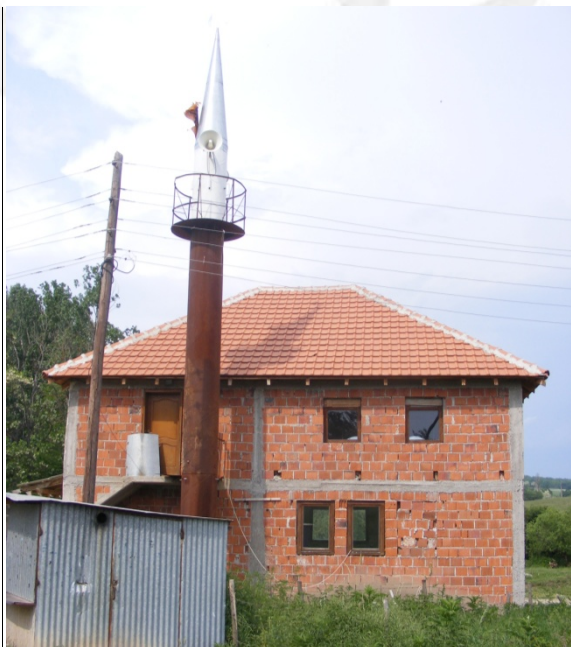
Fig. 1.3 Side facade, south-west
