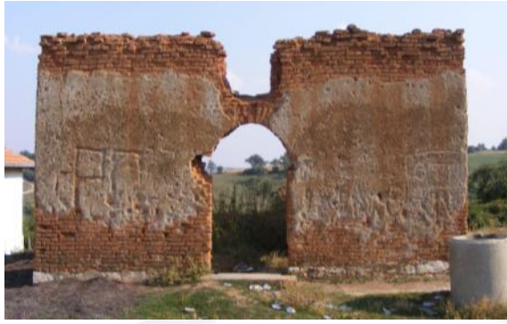
Fig. 1.1 Main / front, north-west facade
