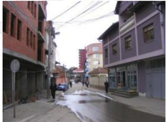
Fig. 1.8 Existing building of lower height in the neighbourhood of the KARAMANLI Mosque to north-west
