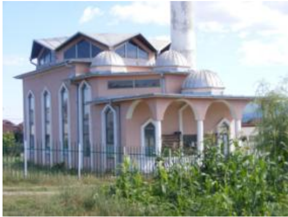
Fig. 4.2 View from the northern side
