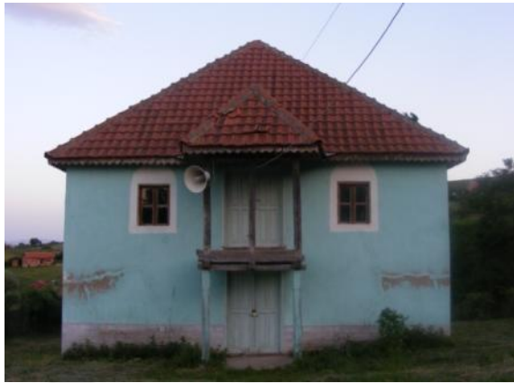
Fig. 1.1 Main / front, north-west facade
