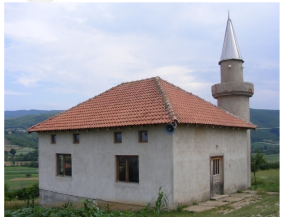
Fig. 1.7 Side facade, north-east
