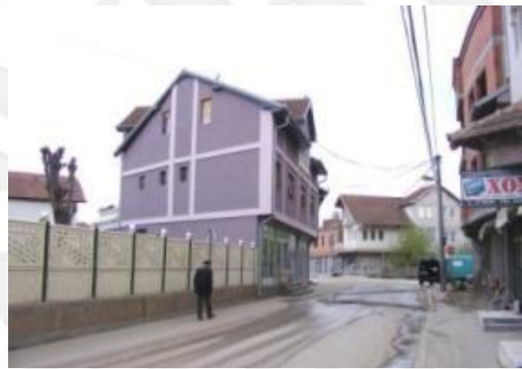
Fig. 1.3 Street that boarders teh parcel of the KARAMANLI Mosque to the west.
