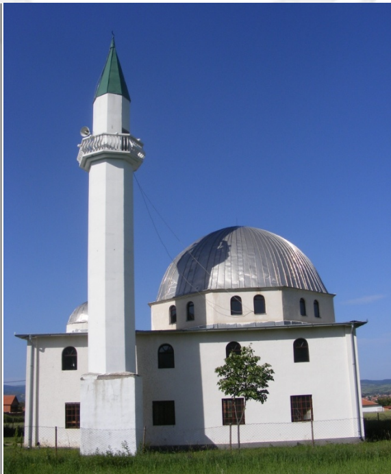
Fig. 1.3 Side facade, south-west
