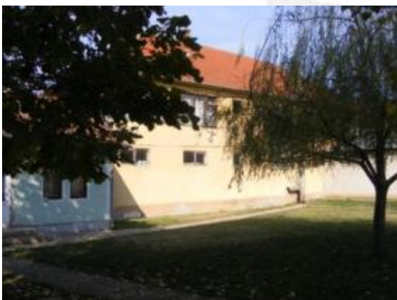
Fig. 2.5 View from north
