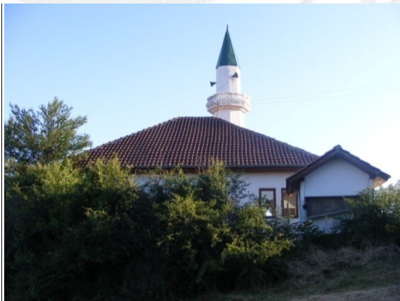
Fig. 1.7 Side facade, north-east
