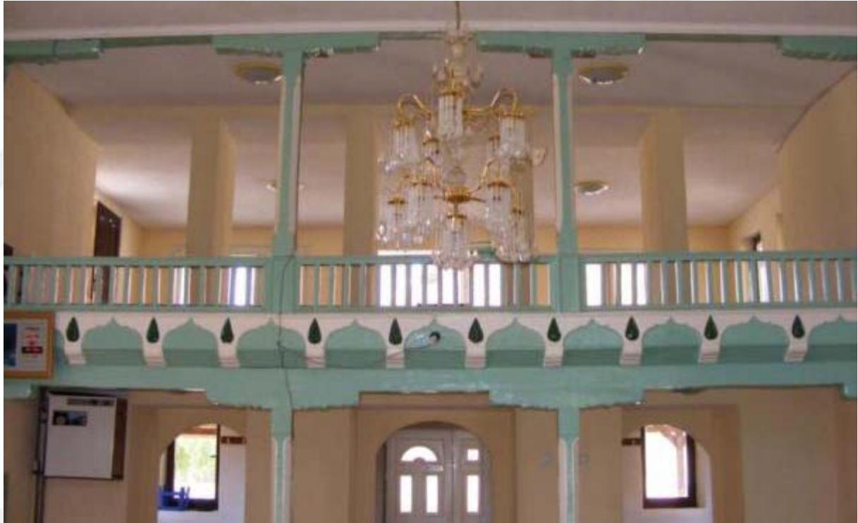
Fig. 1.20 Interior view: the typical piles with bolsters of the Kosovo folk workman. The front of the slab is decorated with relieves (the characteristic arch of the Islamic/ottoman architecture) and the wooden fence.
