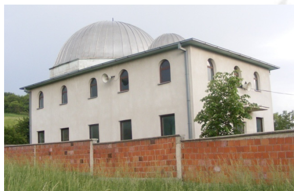
Fig. 1.8 View from north
