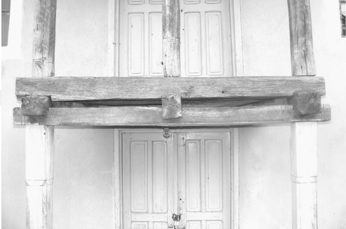
Fig. 3.6 View of the çardak construction.
