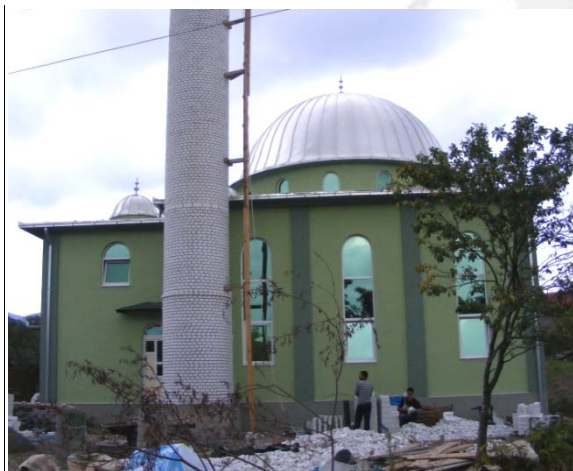
Fig. 1.3 Side facade, south-west
