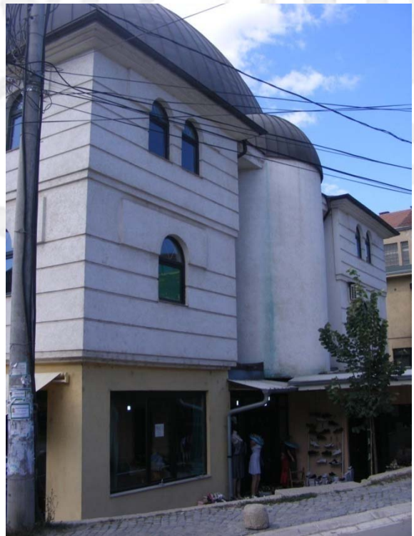
Fig. 1.4 Back façade, southeast
