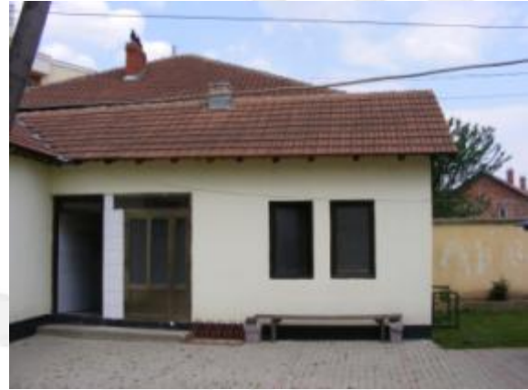
Fig. 2.2 View from north-east.
