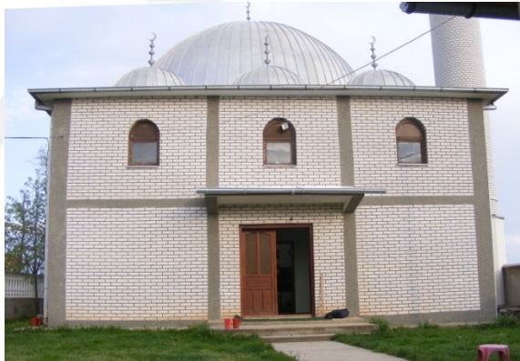
Fig. 1.1 Main / front, north-west facade
