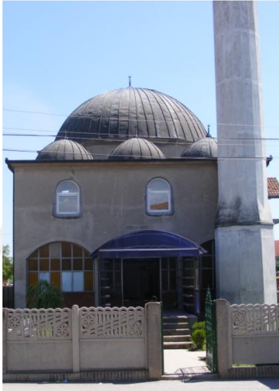
Fig. 1.1 Front/main facade, north-west
