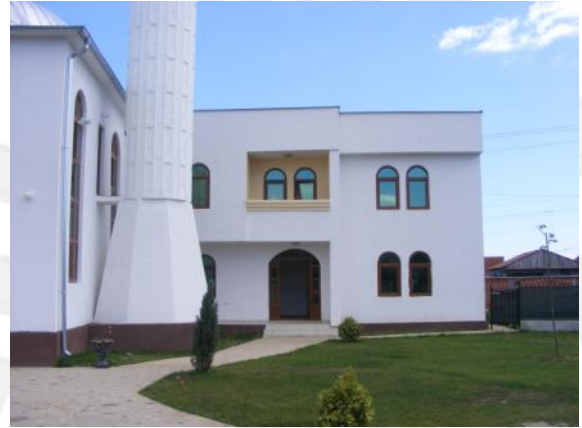
Fig. 1.6 The annex, facade from north-west
