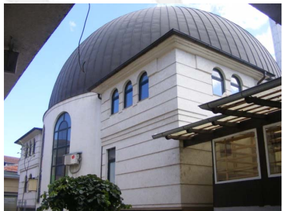
Fig. 1.8 View from north
