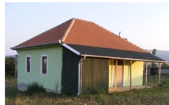
Fig. 1.8 View from north
