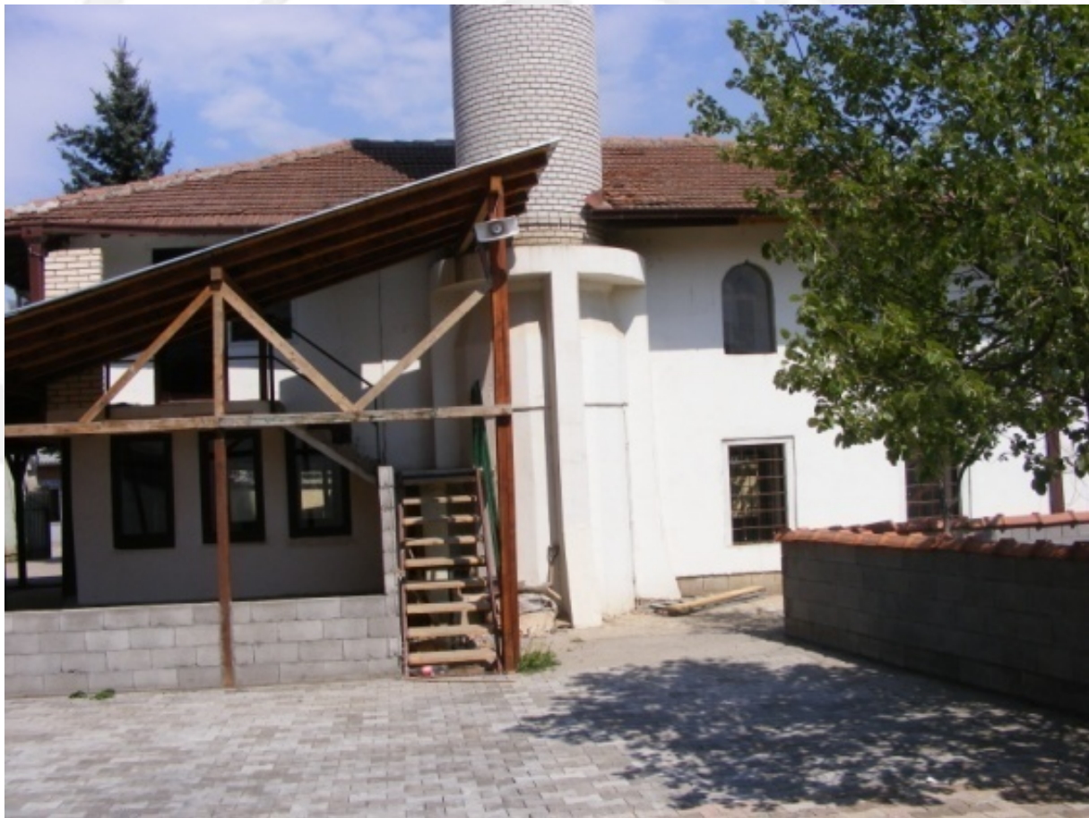
Fig. 1.1 View from the south-west façade.
