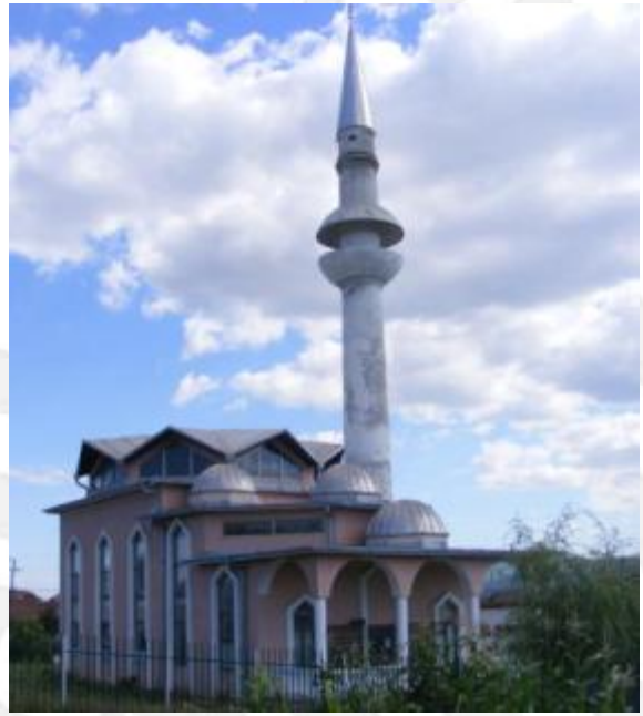
Fig. 1.6 View from the north
