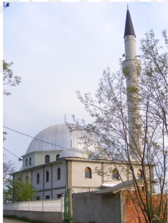
Fig. 1.8 Side facade, north-east
