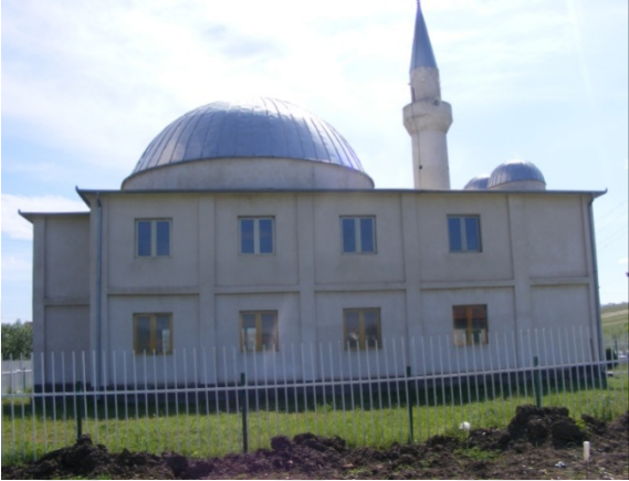
Fig. 1.7 Side facade, north-east
