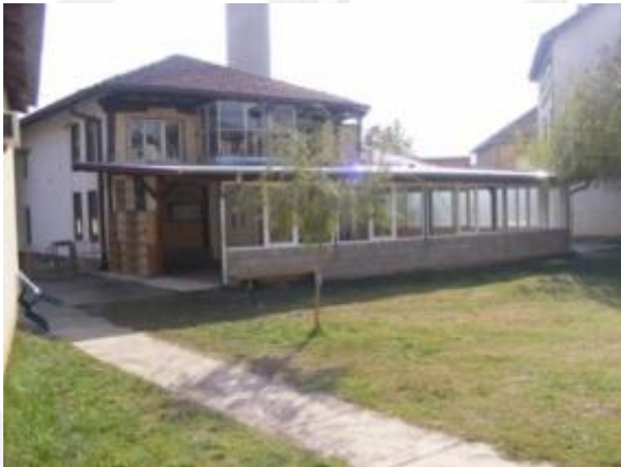
Fig. 2.3 View from south-east
