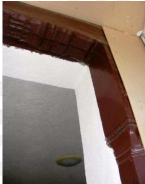
Fig. 1.26 Interior detail – upper floor, the bolster and the pile
