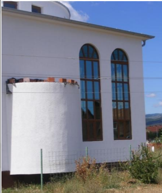
Fig. 6.4 View of the back facade, notice the mihrab without a covering
