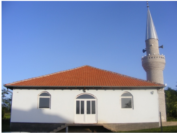
Fig. 1.1 Main / front, north-west facade
