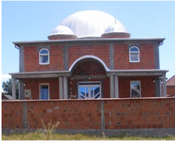
Fig. 1.1 Front/main facade, north-west
