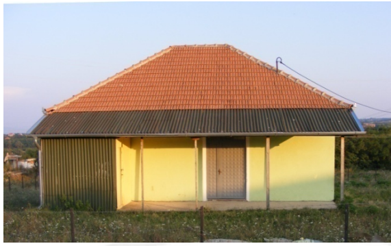
Fig. 1.1 Main / front, north-west facade
