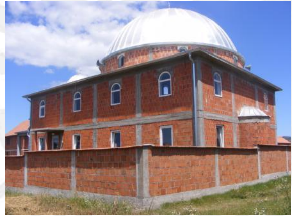
Fig. 1.4 Facade from south
