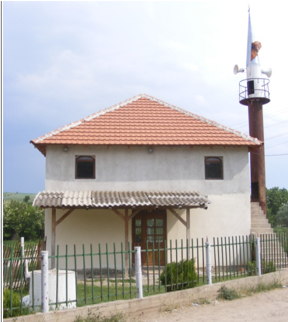
Fig. 1.1 Main / front, north-west facade
