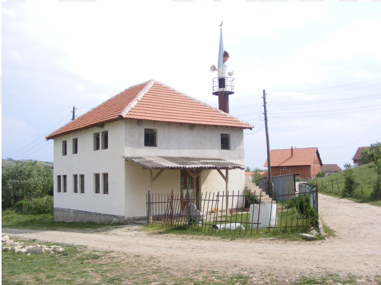
Fig. 1.7 View from north
