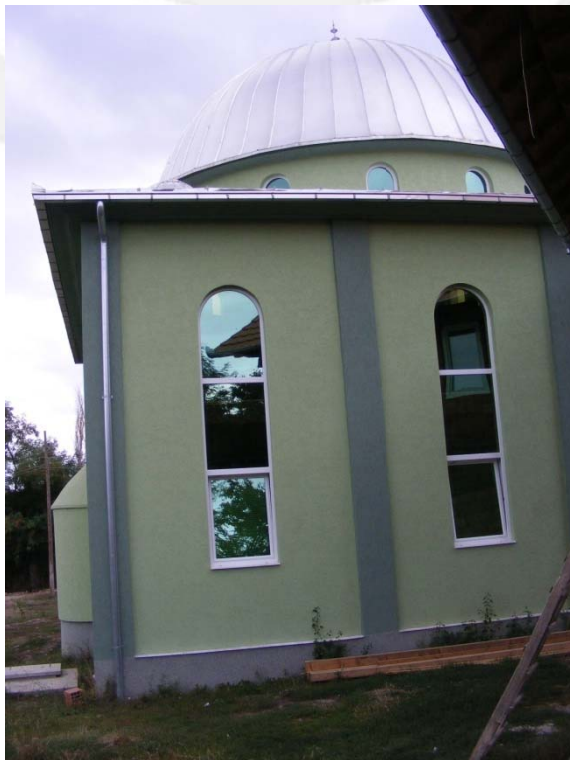
Fig. 1.7 Side facade, north-east
