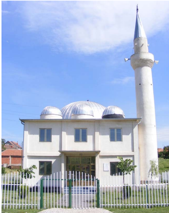
Fig. 1.1 Main / front, north-west facade
