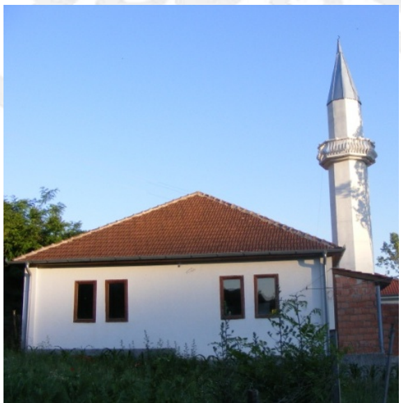
Fig. 1.6 Side facade, north
