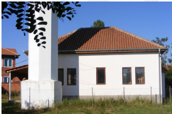
Fig. 1.3 Side facade, south-west
