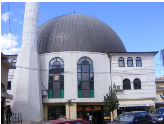
Fig. 1.3 Side facade, south-west
