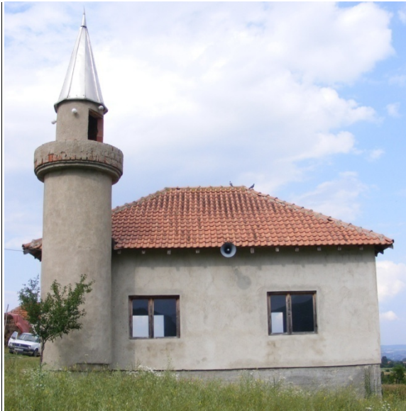
Fig. 1.2 Side facade, south-west
