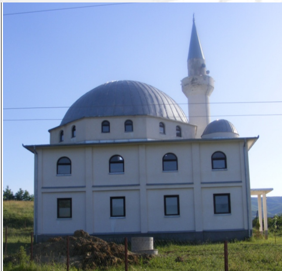
Fig. 1.7 Side facade, north-east
