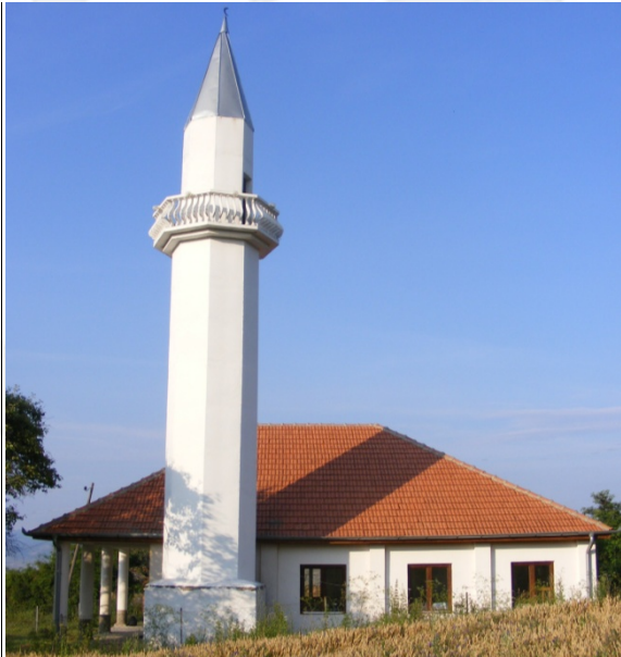
Fig. 1.3 Side facade, south-west
