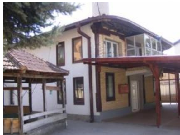
Fig. 3.9 View from north
