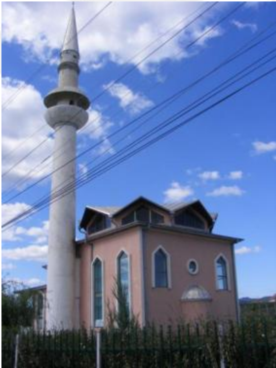
Fig. 1.3 View from the south
