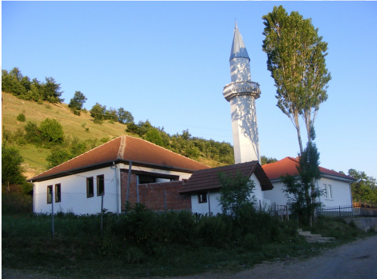
Fig. 13.1 (1.7) View from north
