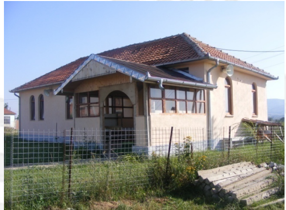
Fig. 1.2 View from north
