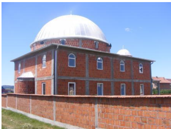
Fig. 1.5 Facade from east
