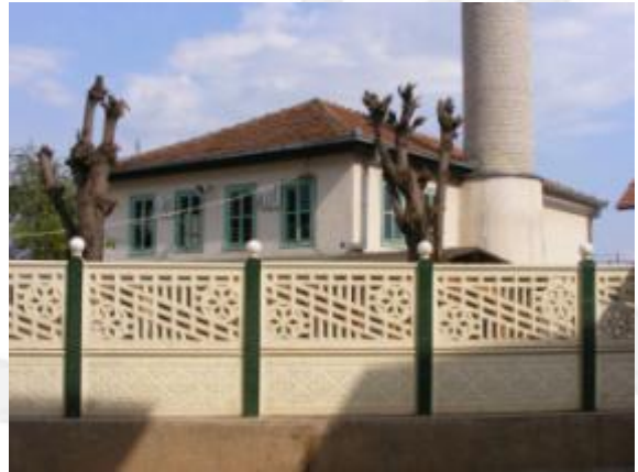
Fig. 3.1 View from north-east
