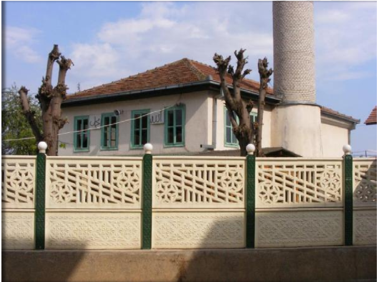
Fig. 2.1 View from north-east
