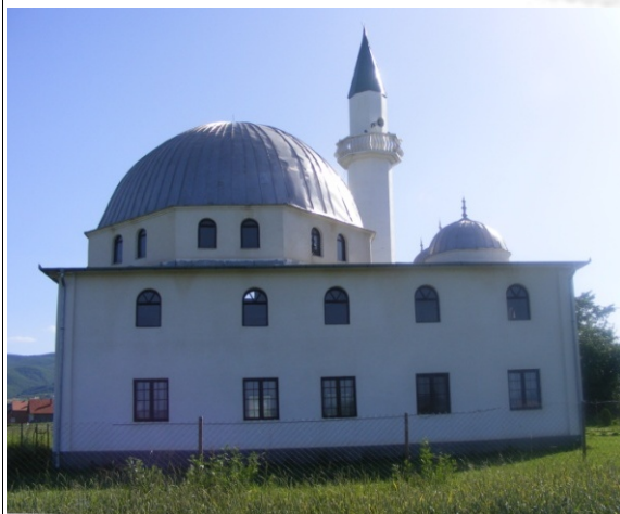
Fig. 1.7 Side facade, north-east
