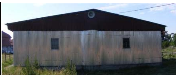
Fig. 1.3 The facade from south-east
