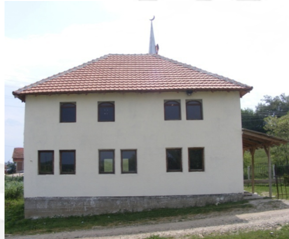
Fig. 1.6 Side facade, north-east
