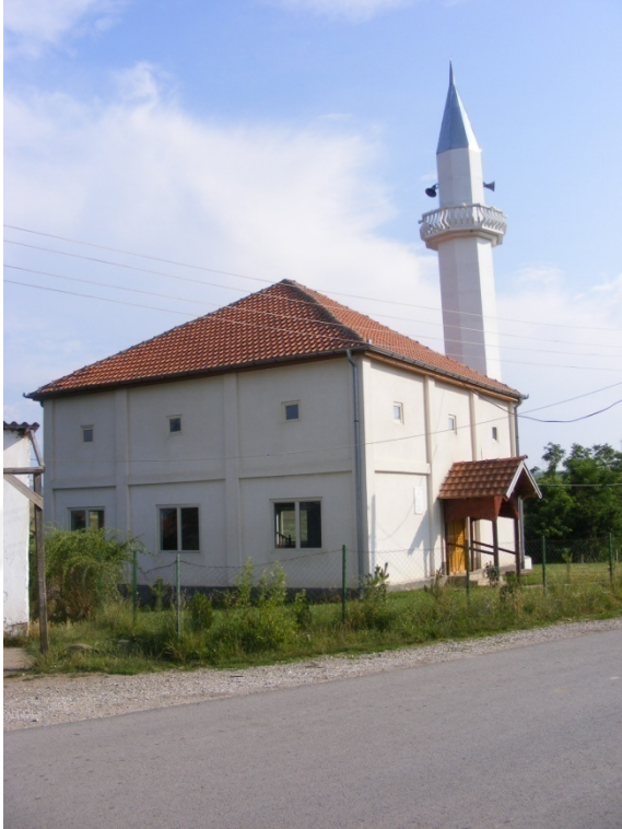
Fig. 1.5 View from north-east
