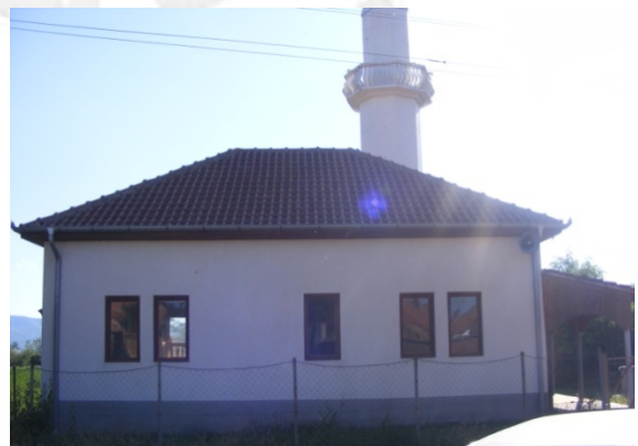
Fig. 1.6 Side facade, north-east
