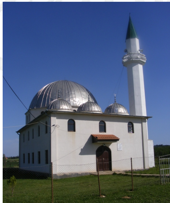
Fig. 1.8 View from north
