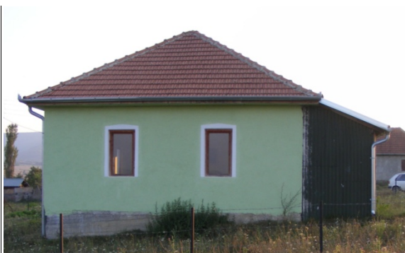
Fig. 1.7 Side facade, north-east
