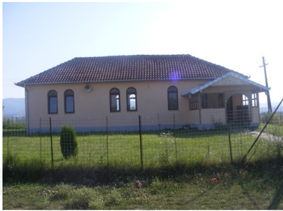
Fig. 1.1 Main / front, north-east facade
