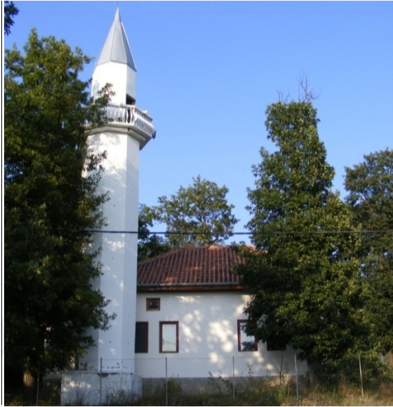
Fig. 1.3 Side facade, south-west
