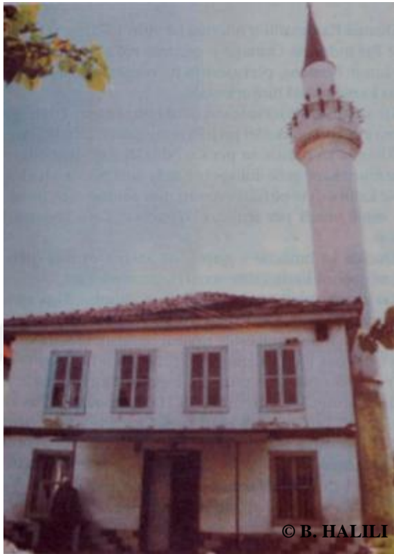
Fig. 2.7 View from north-west, picture from before the war (1999). This Minaret does not exist today.
