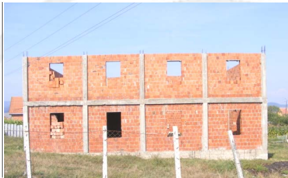
Fig. 1.3 Side facade, south-west
