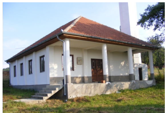
Fig. 1.6 Side facade, north
