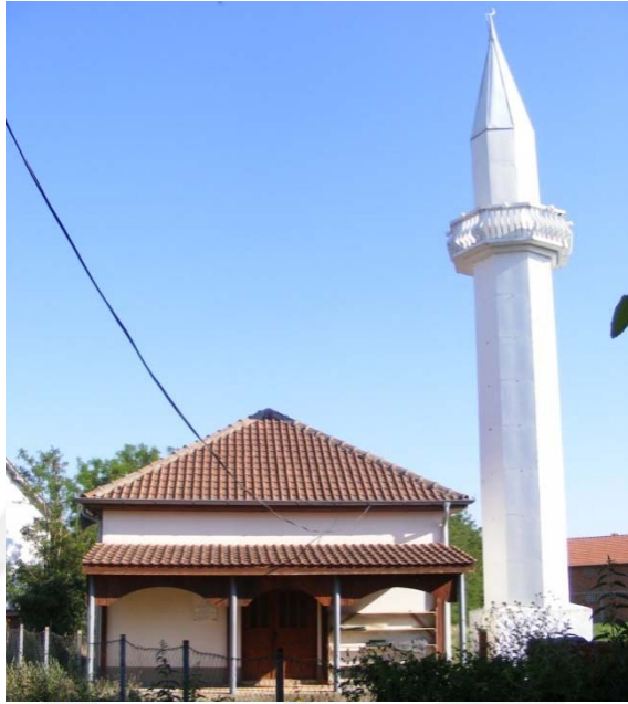
Fig. 1.1 Main / front, north-west facade
