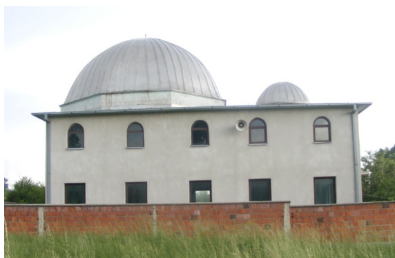
Fig. 1.7 Side facade, north-east
