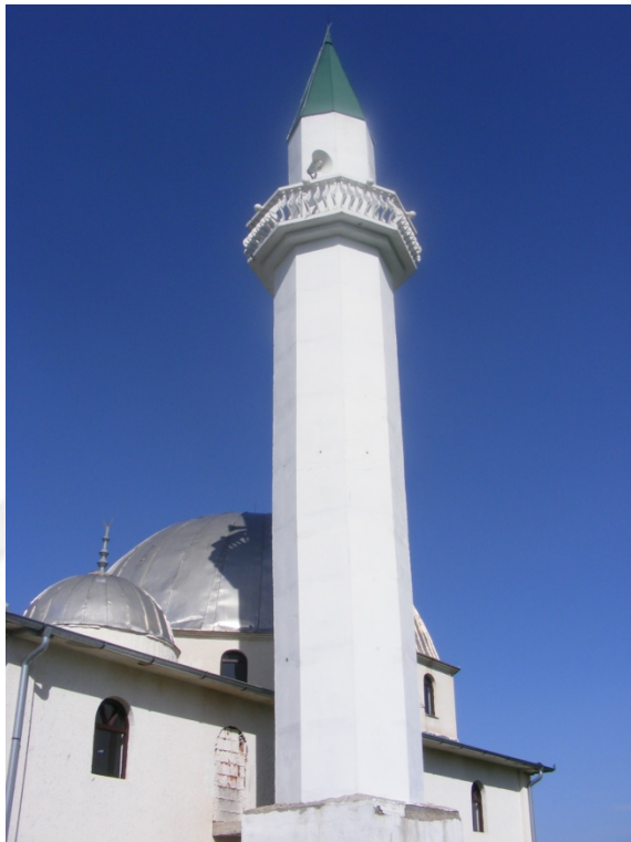
Fig. 7.2 Minaret, view of the covered door sherife and conic roof
