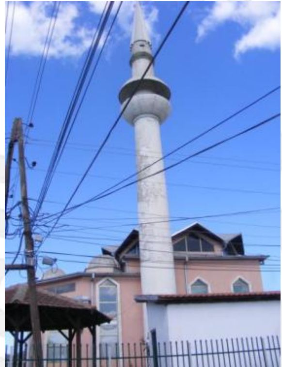
Fig. 1.2 Side facade, south-west
