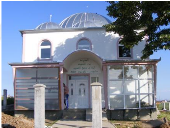
Fig. 1.1 Main / front, north-west facade
