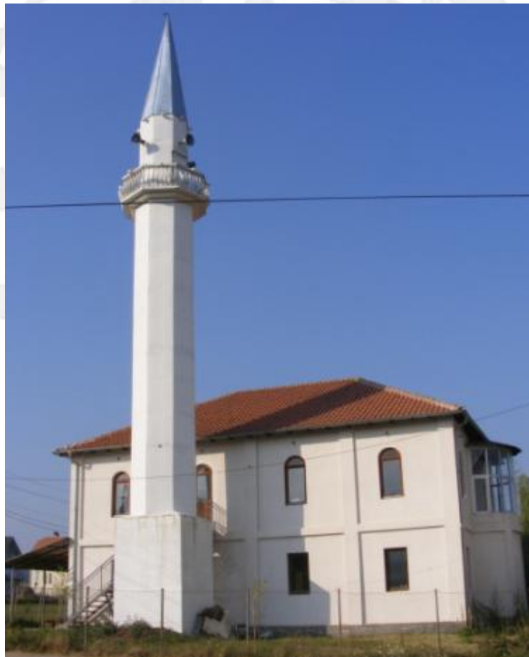
Fig. 5.1 View from south-west
