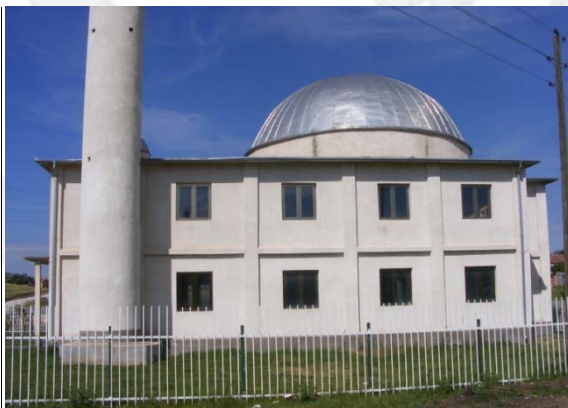
Fig. 1.3 Side facade, south-west
