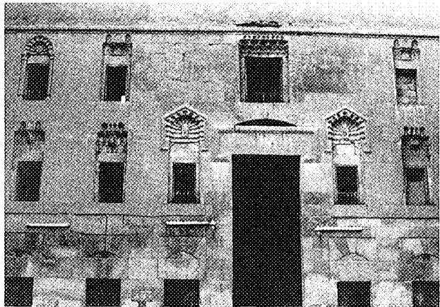
Fig. 7. Khanqah of Baybars. Window of cells opening onto the courtyard.
