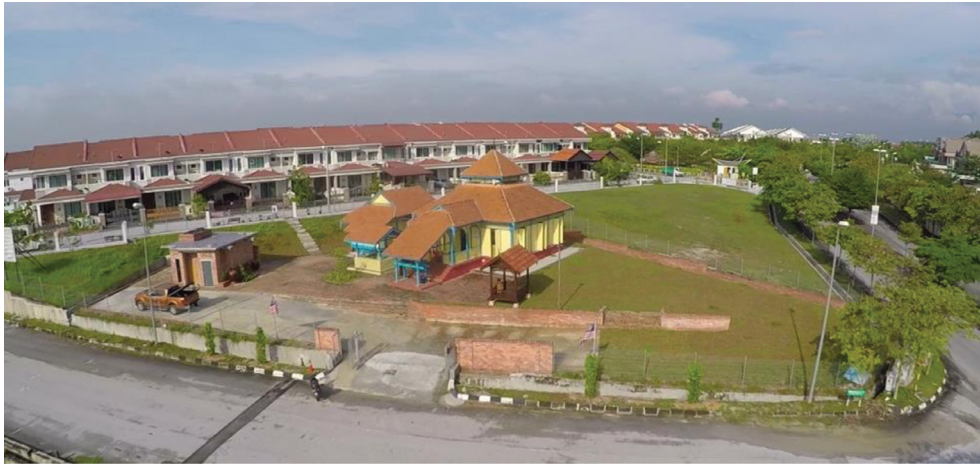
Figure 1: Aerial view of Kampung Teluk Memali Mosque in Ipoh, Perak, Malaysia.
