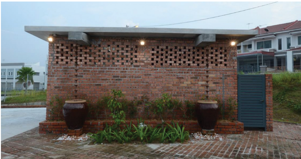
Figure 4: The new toilet building.
