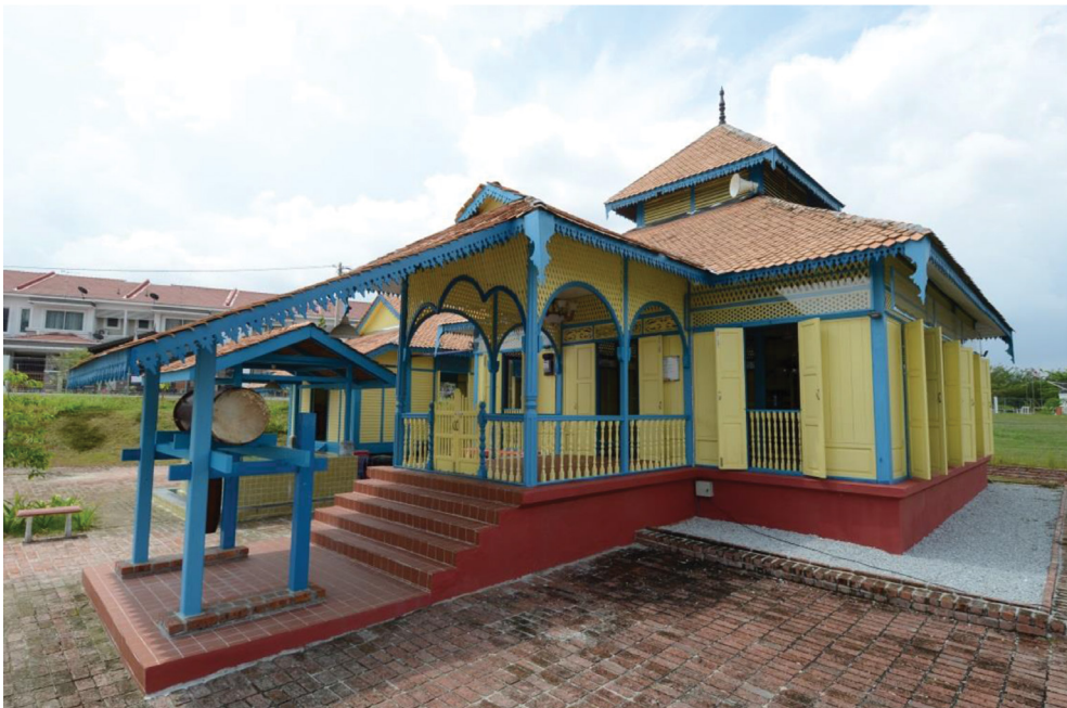
Figure 2: Conditions of mosque building after the completion of conservation works.
