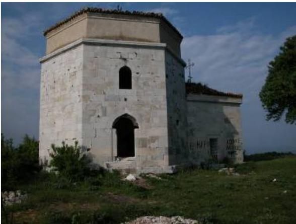
**Lateral view of southern side of monument from the summit on which it is set. Note the fine quality and precision workmanship of the marble facing. Some cracks and missing pieces are evident but, otherwise, the exterior walls have survived the centuries well. The tambour atop the marble walls is made of rubble coated with plaster, a technique that helps us date the monument to the 15<sup>th</sup> century. The tambour was renewed during the restoration of the monument during the late 1960s.**
