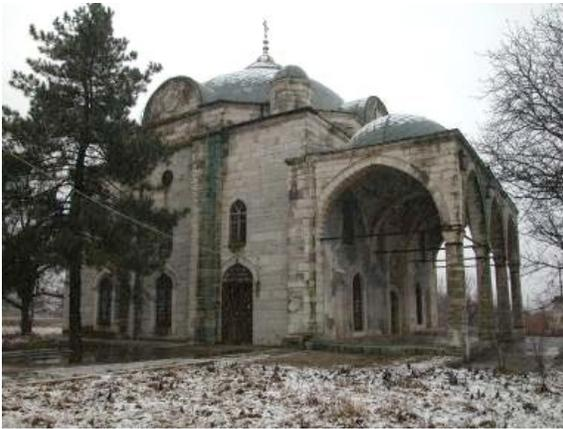
**Oblique view from side. Note the doorway cut into right-most of the three ground-level windows on the left of the building. Also note apparent vulnerability to seepage of buttressing piers on lateral wall.**
