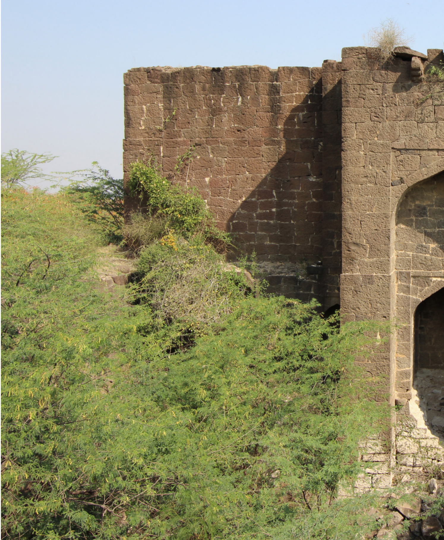
Baoli and hammam located east of Chotta Sarai, built in 1543-1580 CE Location: Shahpur suburb (Bijapur)
