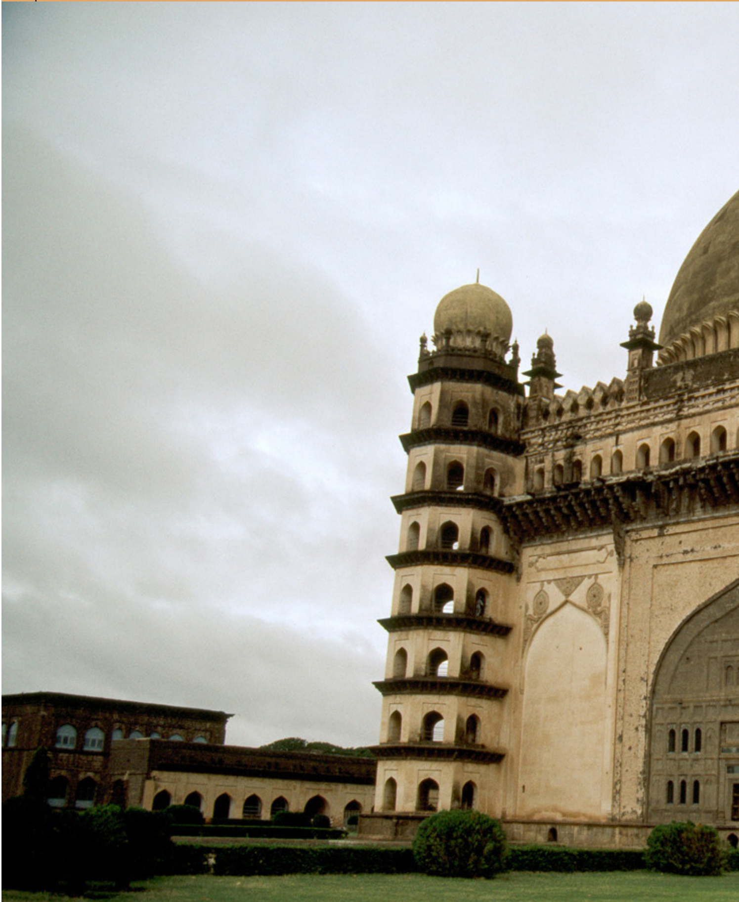
Gol Gumbaz east façade, built in 1627-1656 CE Location: Bijapur, India
