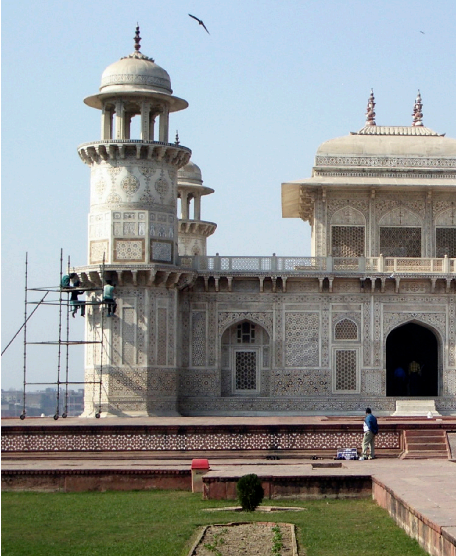
Exterior view of Mausoleum of I'timad al-Daula from the west, built in 1622-1628 CE Location: Agra, India
