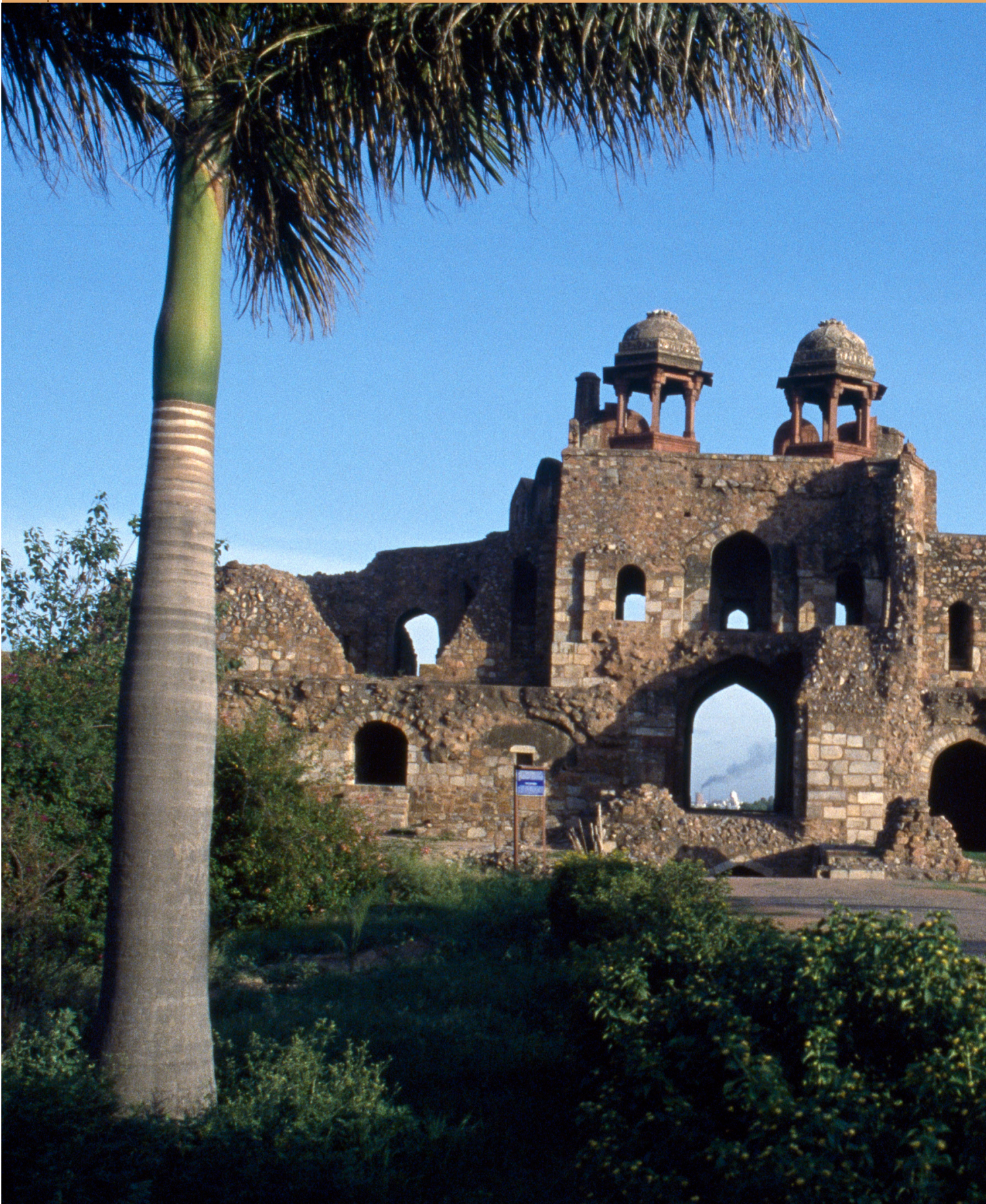
Purana Qil'a, Humayun Darwaza, built in 1543-1544 CE Location: Delhi, India
