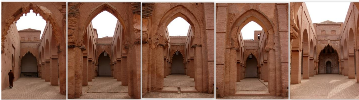
Figure 1.3. Hierarchical Arch Distribution, Side Aisle (left) to Mihrāb (right), Tinmal Mosque (Collage of Author's Photos)
