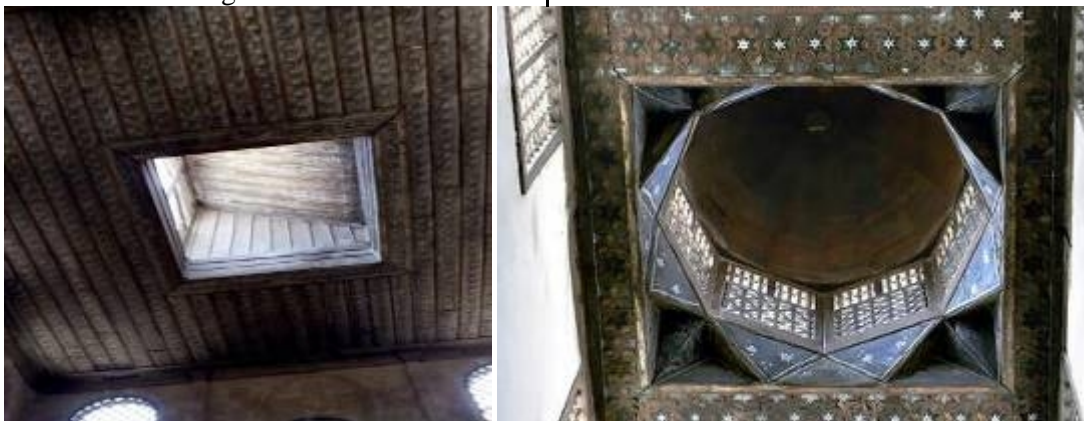
Figure 3: wind tower in Zainab Khatoon house(right) and malqaf in Soliman Agha mosque(left)
