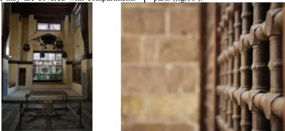
Figure 16: mashrabiya was a good solution in Islamic houses for preventing direct sun rays through it's wood cutting
