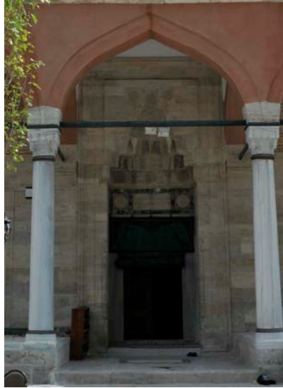
Figure 125: Entrance. Ibrahim Pasha mosque. (Author, 2015)
