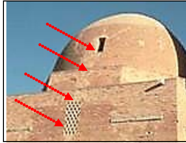
Figure 80: Openings . Bariyan Jameh mosque. (Author, 2015)
