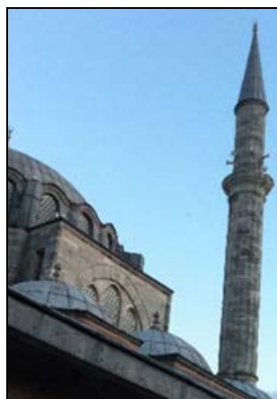
Figure 121: Minaret. Rustam Pasha mosque. (Author, 2015)
