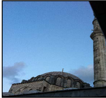
Figure 118: Dome-building. Rustam Pasha mosque. (Author, 2015)
