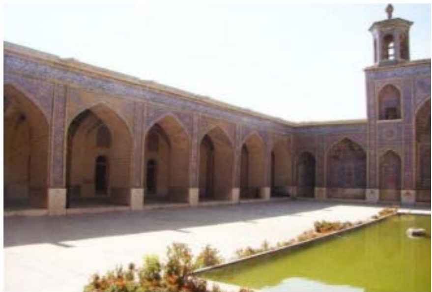
Figure 18. The courtyard eastern wall (Source: author).
