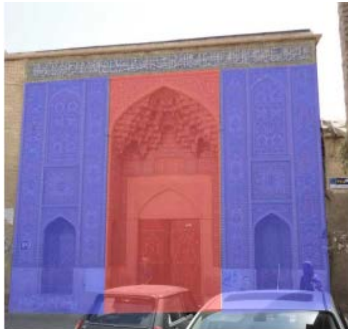
Figure 7. Entrance portal (Source: author).
