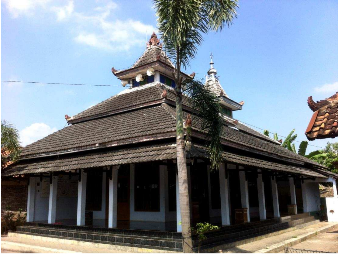
A mosque in Yogyakarta, Indonesia, fully conforming to the prevalent local cultural and environmental demands.
