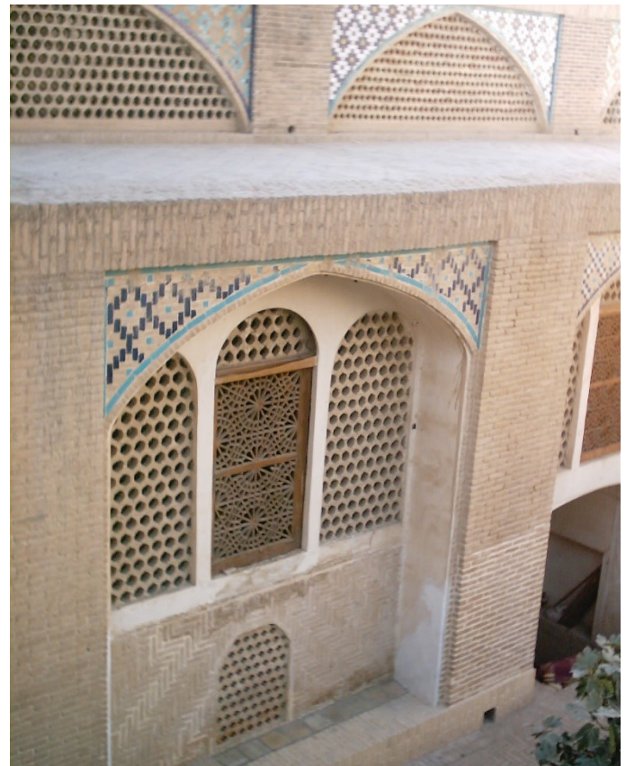
Figure 9: Agha Bozorg Mosque of Kashan; one of the most beautiful examples of window and Shabaak combination. Source: Authors
