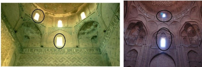
Figure 4: Similarities in the lighting technique of the dome with the Rowzan in the mosques from two different historical periods (right: Jameh Mosque of Isfahan – 5th century A.H. (1009 CE – 1106 CE); left: Jameh Mosque of Varamin – 9th century A.H. (1397 CE – 1495 CE)). Source: Authors
