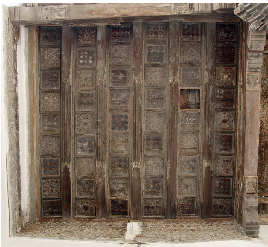
Fig. 22. Paneled ceiling in the southeastern bay of the portico. (Photo: Jasmin Badr)
