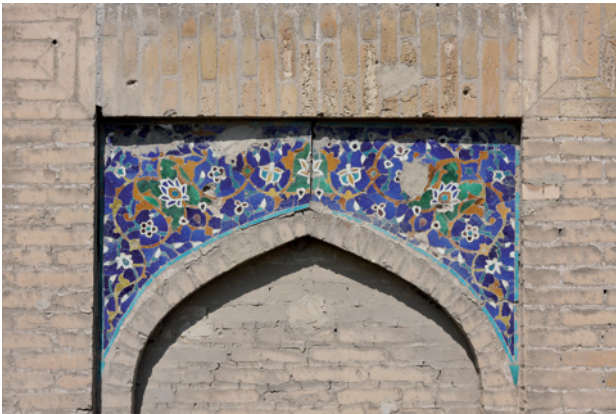
Fig. 6. Tile mosaic in the spandrel of a blind niche in the southern façade of the Khoja Zainuddin Mosque. (Photo: Jasmin Badr)
