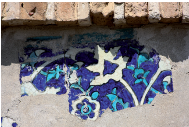
Fig. 7. Underglaze tile in the spandrel of a blind niche in the southern façade of the Khoja Zainuddin Mosque. (Photo: Jasmin Badr)
