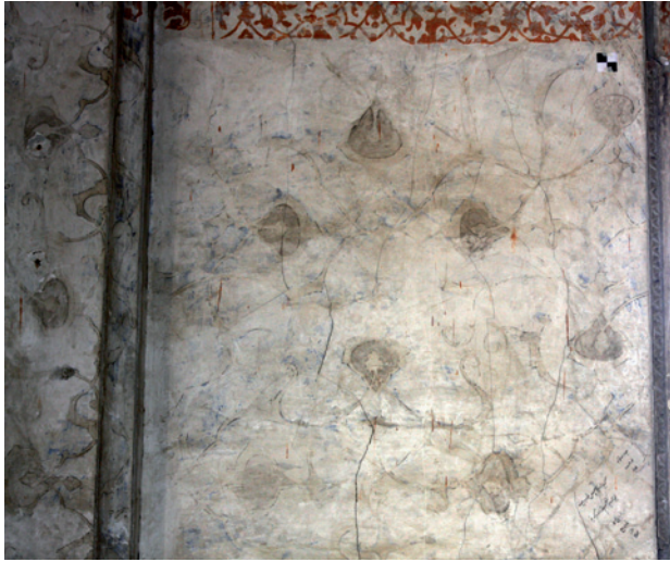
Fig. 17. First decoration phase on the south wall. (Photo: Jasmin Badr)
