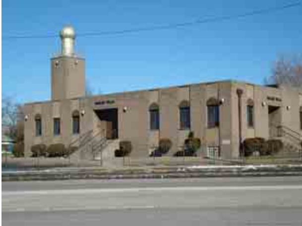
Figure 4.7: Masjid Bilal mosque (Source: Author's photographs).
