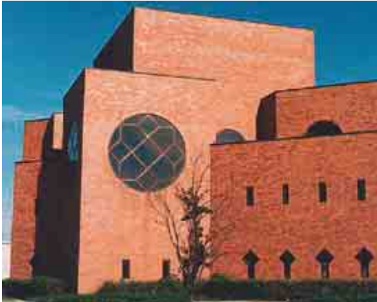
Figure 2.12: Example of innovative design: Islamic Society of North America, Headquarters. Plainfield, Indiana (Khalidi, 2006, 27)
