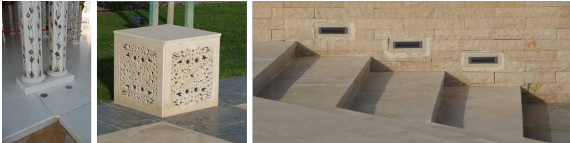
Figure 74: Integrated mosque lighting options.
