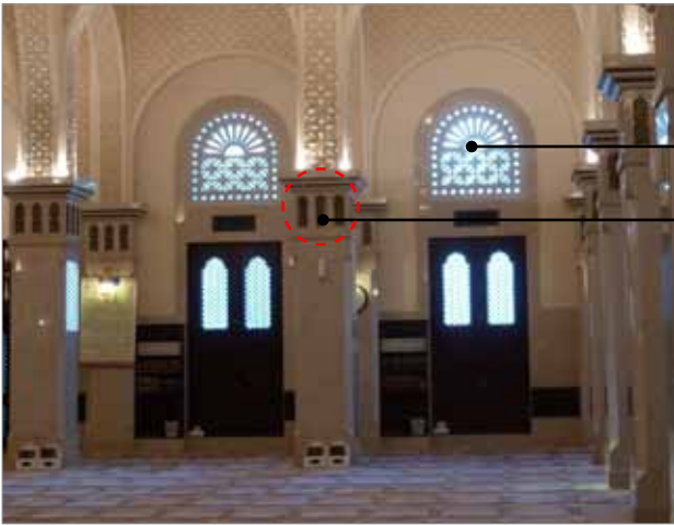
Figure 36: AC vents integrated into the interior design.
