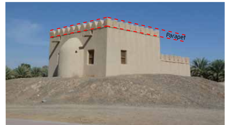
Figure 23: Minimal articulation of the parapet, Hamad Bin Sultan Mosque, Al Ain, UAE.
