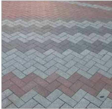
Precast concrete paver: honed finish
