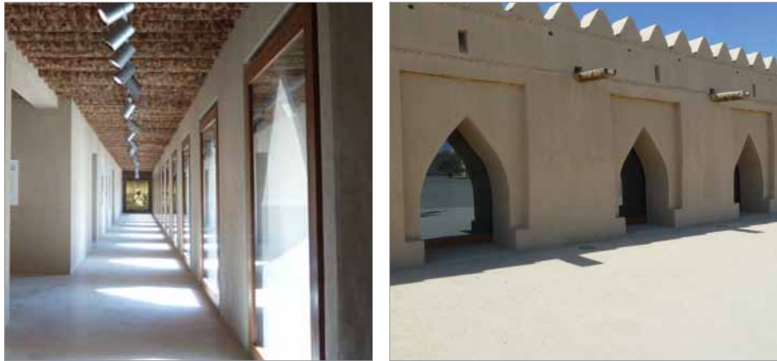
Figure 46: Recessed windows reduce glare, Al Jahili Fort, Al Ain, Abu Dhabi, UAE.
