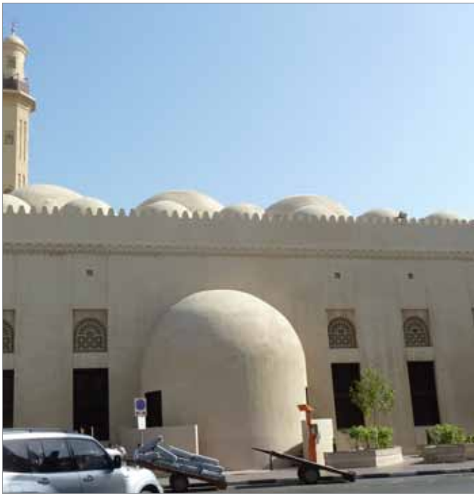
Figure 37: Prominent mihrab on the main prayer hall with entry for Imam, Dubai Grand Mosque, Dubai, UAE.
