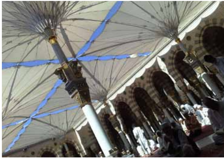
Figure 39: Example of sahan shading, The Prophet's Mosque, Medina, the Kingdom of Saudi Arabia (KSA).
