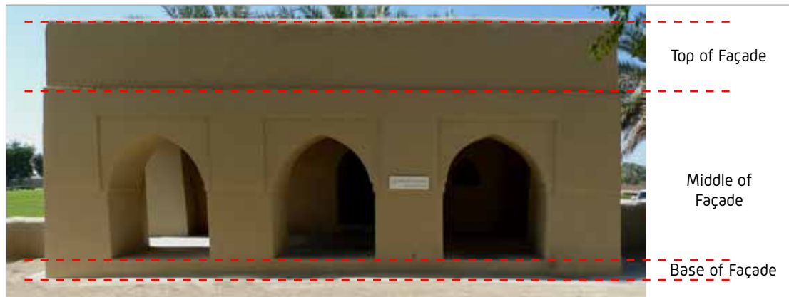
Figure 22: Subtle articulation of base, middle and top of Al Jähili Mosque, Al Ain, UAE.
