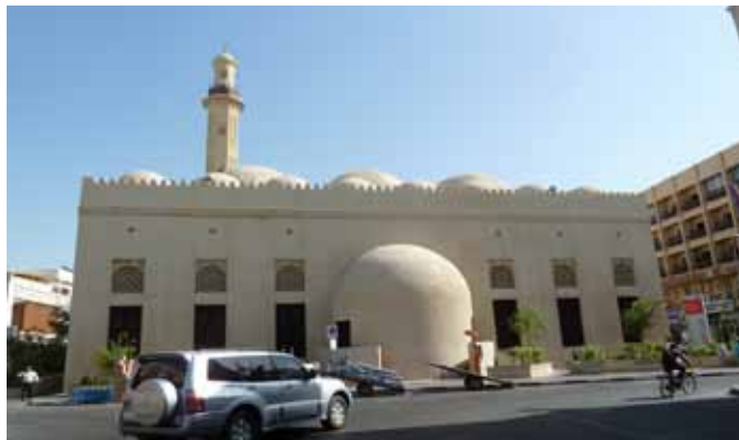
Figure 27: Unobtrusive domes to create an internal ambience, Grand Mosque, Dubai, UAE.
