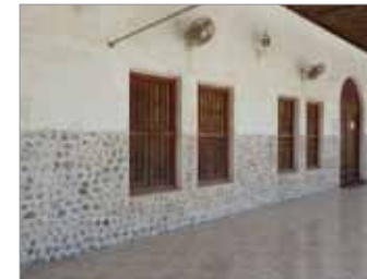
Figure 51: Rubble and gypsum texture, The National Museum of Ras Al Khaimah, UAE.
