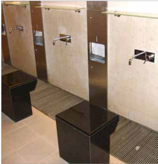
Figure 44: Abluion design with splash-free grating and without a step.
