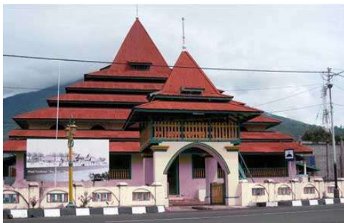
a. STM Building in front of.
