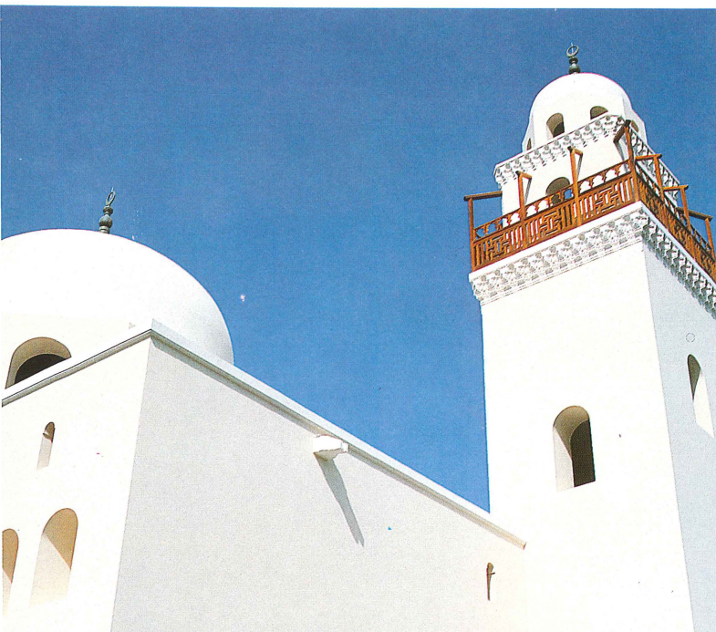
Below: View of the minaret with a wooden balustrade and the mosque at the left. Below, right: Ground floor plan. Far right: View of the main entrance door.
