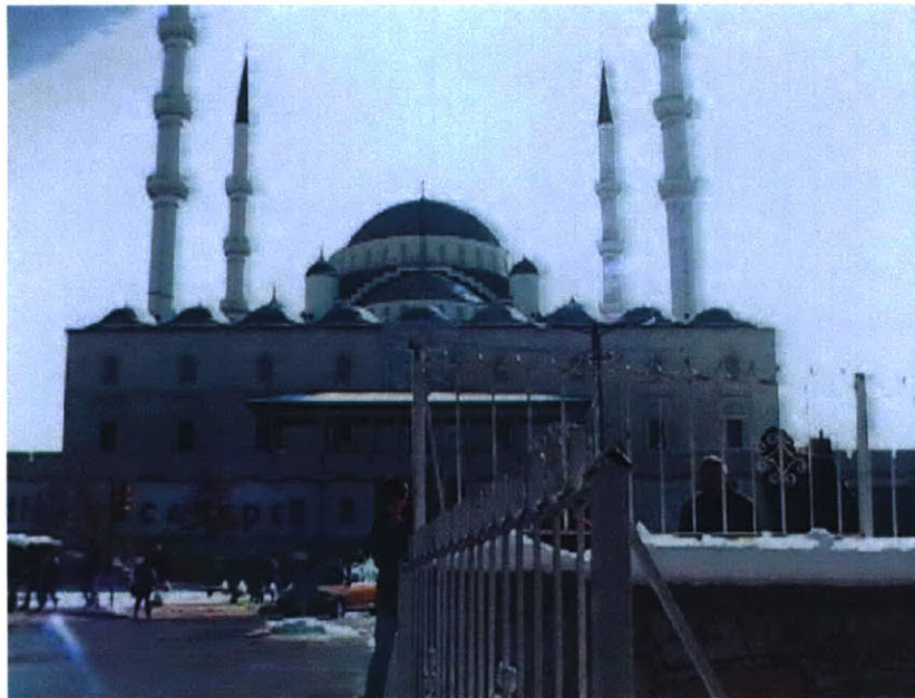
Fig.46 Approach from the from the north.
