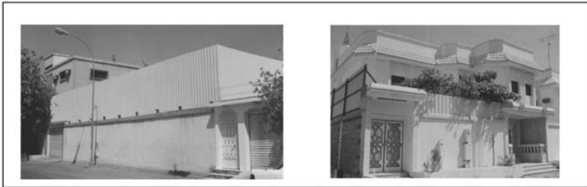
Fig. 2.13. Two villas in Hofuf (people altered the façades of their houses to provide more privacy for the front setbacks by using metal sheets to increase the height of their house fences). Source: Visual survey 1995.
