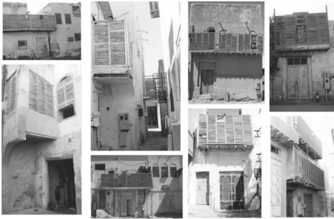
Fig. 6.18. External agasi linking the majlis upstairs with the main sikka . Source: Author.
