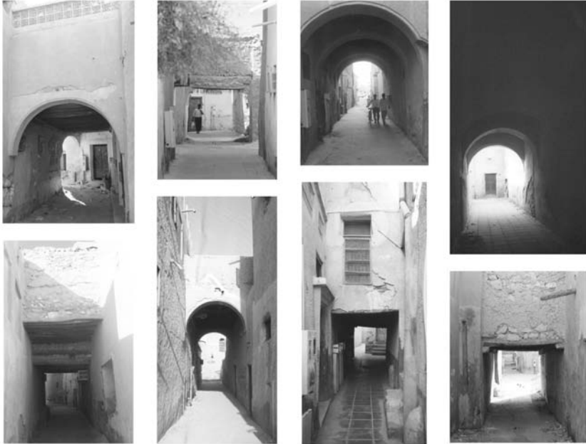
Fig. 5.17. Sabats in the traditional home environment had worked as connection elements which bound the fereej physically. Also they created a contrast between shade and light and provided places for old men and children to enjoy themselves in the external domestic spaces in a hot arid climate. Source: Author.
