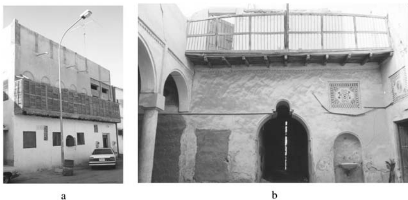
Fig. 6.30. The agasi . a) External agasi associated with the male reception spaces upstairs. b) Internal agasi looking over the courtyard. Source: Author.
