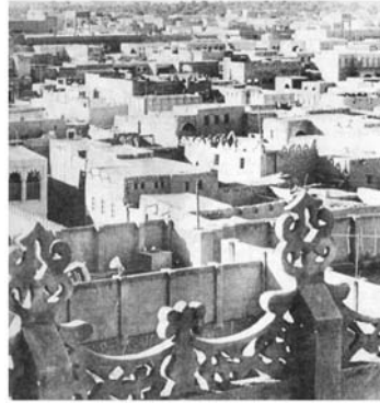
Fig. 5.18. A view taken from the old Emirate building in the northern part of Alkut shows the mass of the first floors. They had always formed the main façade of the house to protect the family zones and to let the members of the community use their roofs freely. Also, they express a symbolic meaning by connecting the men's reception spaces with external domestic spaces. Source: Aramco.
