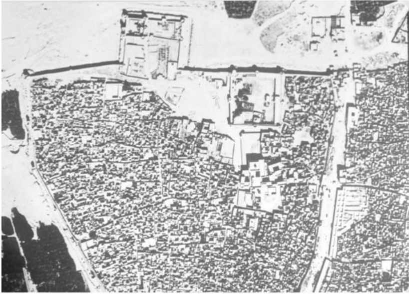
Fig. 5.3. Unitary physical mass of the traditional neighbourhood ( Alkut and part of the northern Arrifa ). It is impossible to define the hidden boundary of the fereej system. Source: Aramco.
