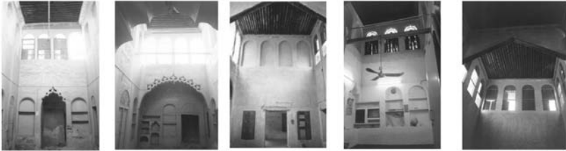
Fig 6.9. Majlis of two storeys. Usually it was ventilated and lighted through a number of windows facing north and some time south and east. The coffee place was usually situated in the front zone of the majlis hall. Source: Author.
