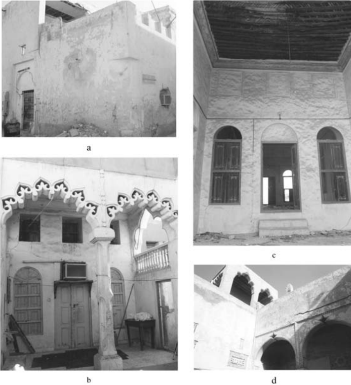
Fig. 6.16. The masbah in the traditional house took several forms and locations. a) The masbah seen from the main sikka to indicate the majlis upstairs. b) Two decorative arches opened to guest roof in the majlis masbah . c) High roof masbah to indicate the majlis from outside and to emphasise the importance of the majlis . d) Masbah in the family part looking to the family courtyard. Source: Author.
