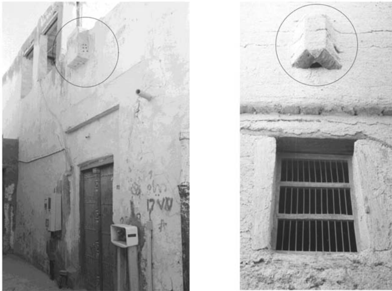
Fig. 5.28. Openings in the tarma used by women to observe the external domestic space.
