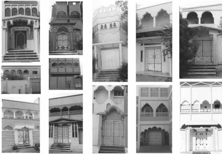
Fig. 2.1. A number of villas constructed in 1980's and 90's influenced by the image of traditional loggia in the main façade. Source: Author.
