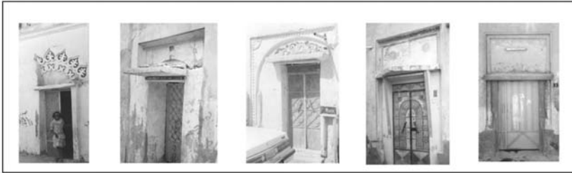
Fig. 2.7. A number of traditional house gateways transformed to imitate the new house types in 1950s and 60s in Hofuf. Source: Visual survey 1995.
