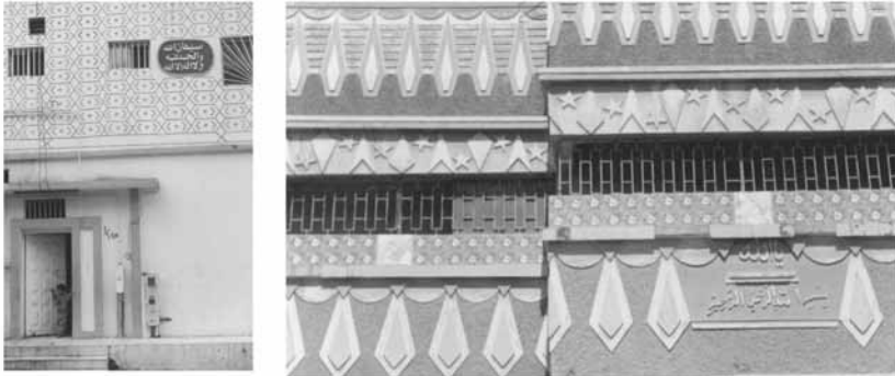
Fig. 1.35. The cement plastered used as a decoration medium to personalise the house. Source: Author.
