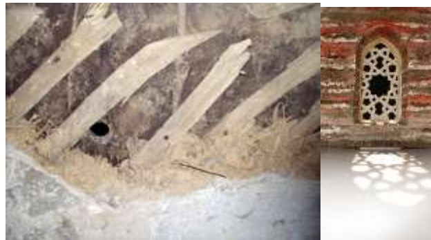
Fig. 17. (Left) earth and wooden lattices used as finishing material in vernacular architecture in Kosovo. (Right) study model of rammed earth wall and window as an atmospheric space. Source: Author's photo courtesy
