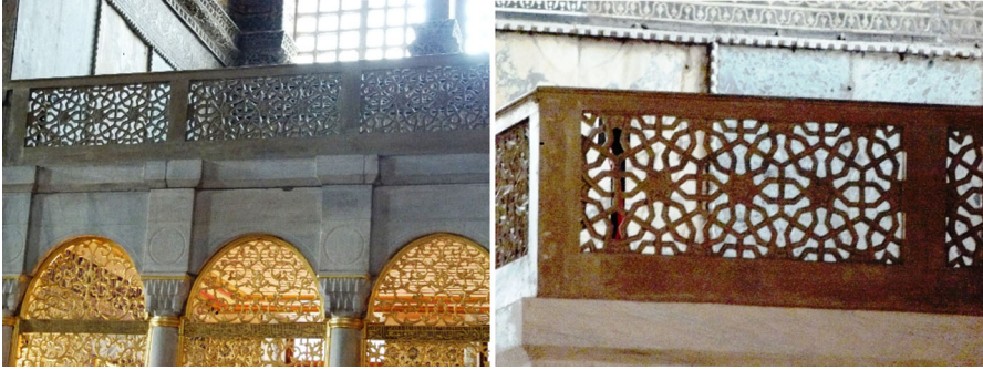
Fig. 4 a Left the Library of Sultan Mahmud I, Hagia Sophia; b right detail of the grill on the upper level. Photos: authors
