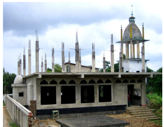
Fig: 17: Vertical extension with permanent structures.
