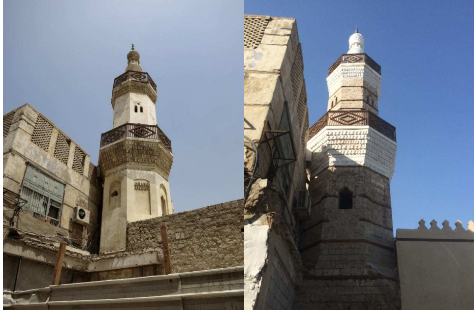
Fig. 26: Al-Shafi'i Mosque Minaret, Before and After Recent Restoration
