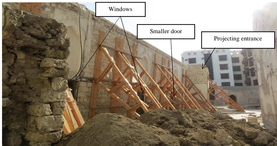
Fig. 9: Al-Shafi'i Mosque Exterior Northern Wall
