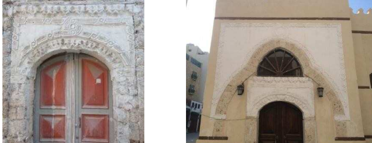
Fig. 6: Al-Shafi'i Mosque Small Door on the Southern End of the Qibla Wall, Before and After Recent Restoration
