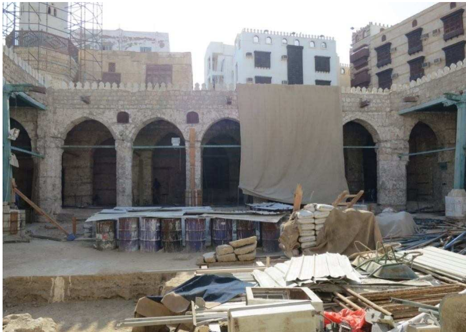
Fig. 25: Al-Shafi'i Mosque Southern Wall
