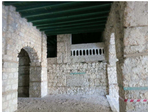
Fig. 14: Al-Shafi'i Mosque Enclosures on the Western Riwaq
