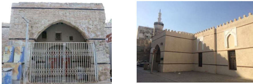
Fig. 7: Al-Shafi'i Mosque Southern Wall, Main Entrance Before and After Restoration. The Entrance's Projection is Shown in the New Picture
