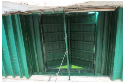
Fig. 22: Al-Shafi'i Mosque First Opening in the Ceiling
