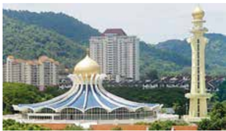
Figure 1: Photo of Penang State Mosque
