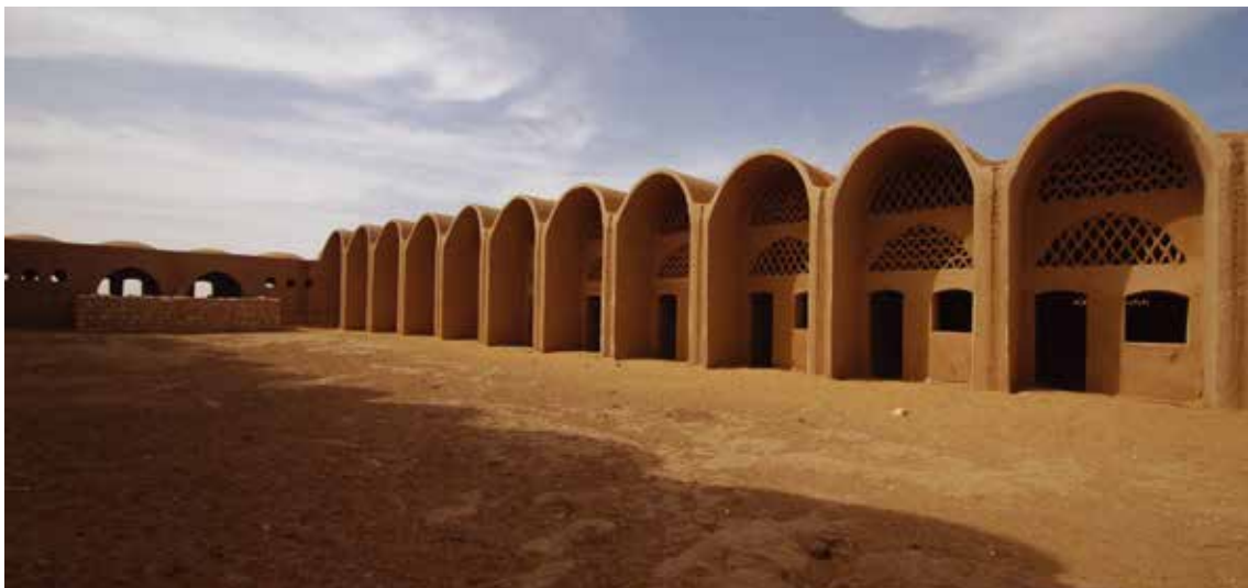
Inner façade of the Market in New Baris. Photo: Zs. Vasáros, 2015.
