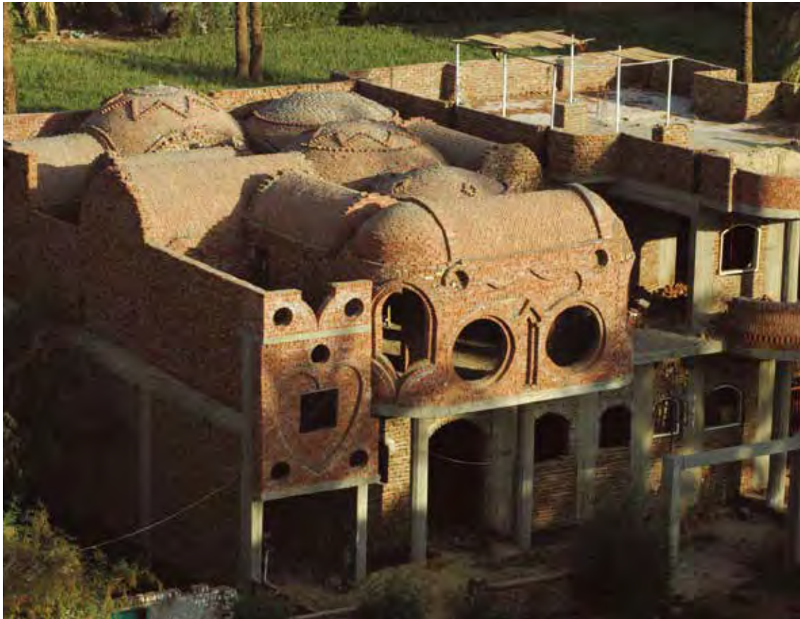
Domed-vaulted architecture in Luxor West Bank. Photo: Zs. Vasáros, 2011.
