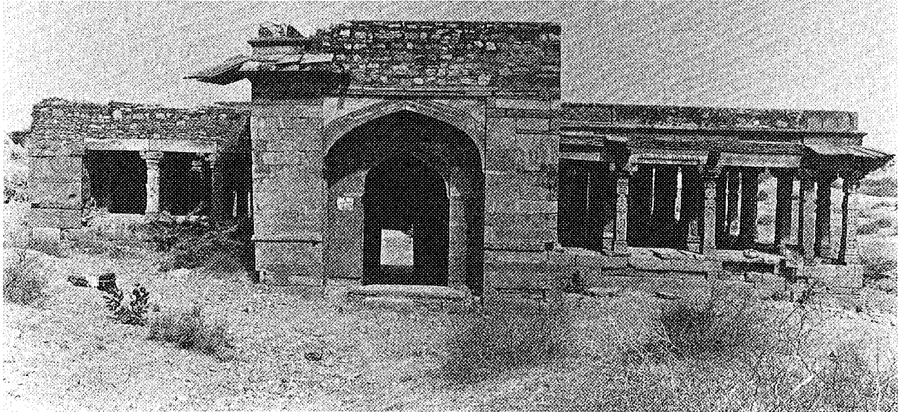
Fig. 5. Kaman, Chaurasi Khamba Masjid. View of the eastern elevation showing main entrance gateway.
