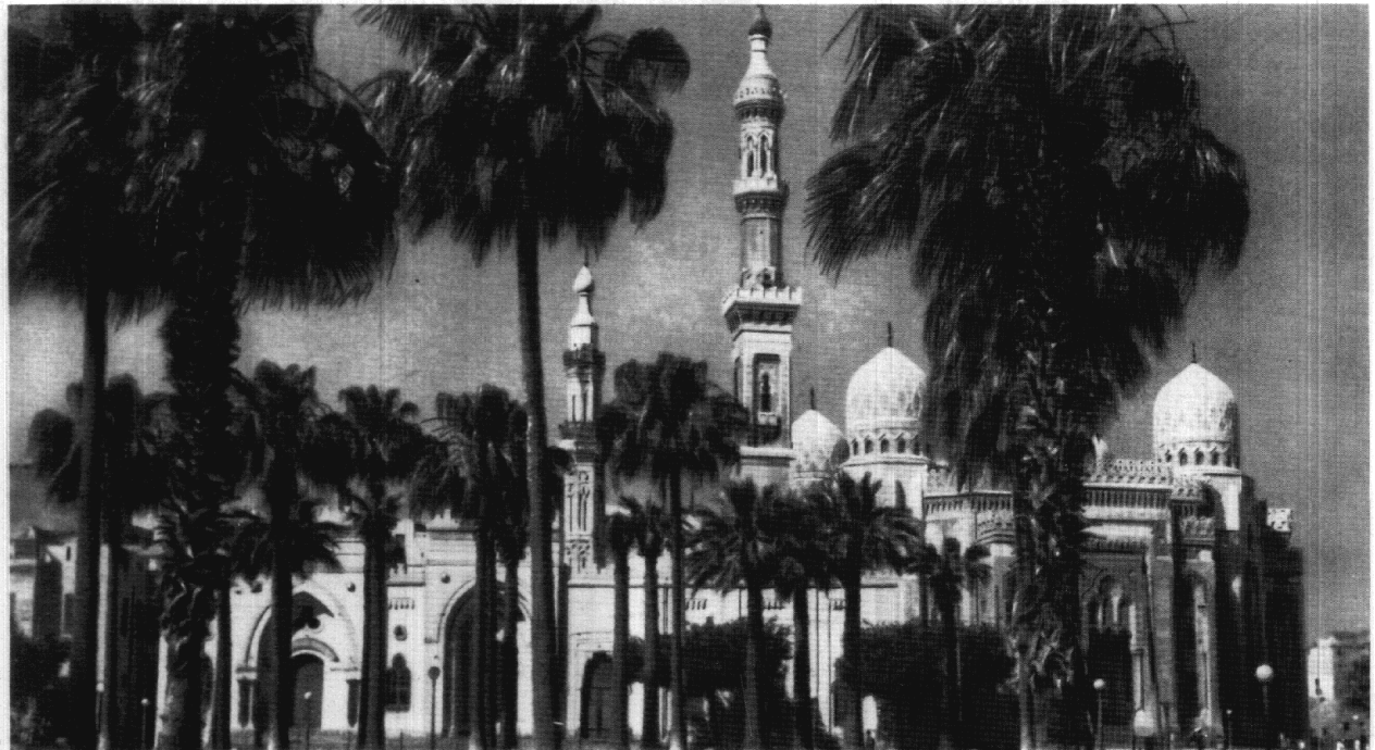
ABU'I-'ABBAS MOSQUE: GENERAL VIEW
