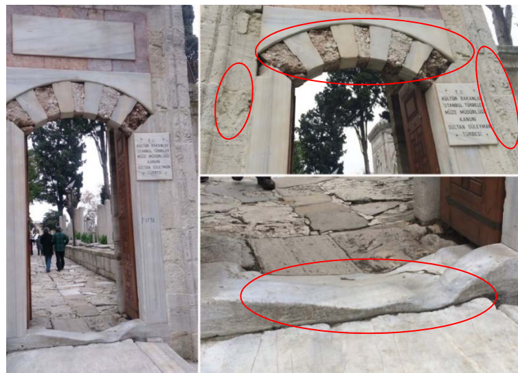
Figure 5. The view of erosion (right up) and abrasion (right down) in Marmara Marble, Hereke Pudding and Küfeki Stone
