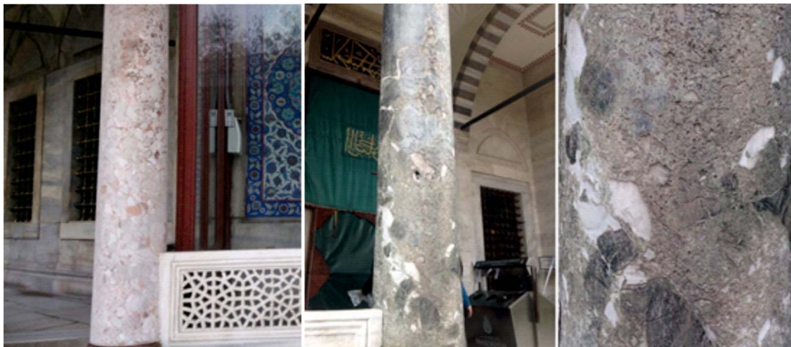
Figure 9. The lose colour of stone in Serpentine Breccia (left) and Hereke Pudding (right)
