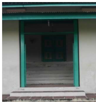
c. Main Entrance
