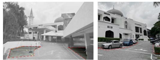
Figure 11. (a) Private parking and (b) Public parking in Saidina Abu Bakar As Siddiq Mosque (Author)
