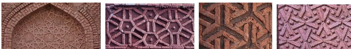
Fig. 5 Tower of Kharaqan in Qazvin, 12-point, 6-point, abstract 6-point, and 8-point geometrical patterns.
