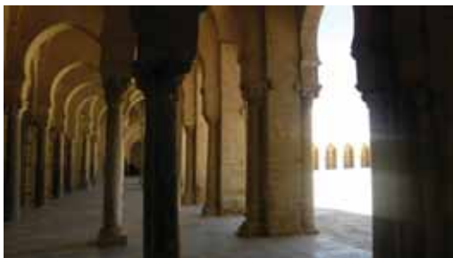
Figure 3: Interior view of the galleries. Source: (Author 2013)
