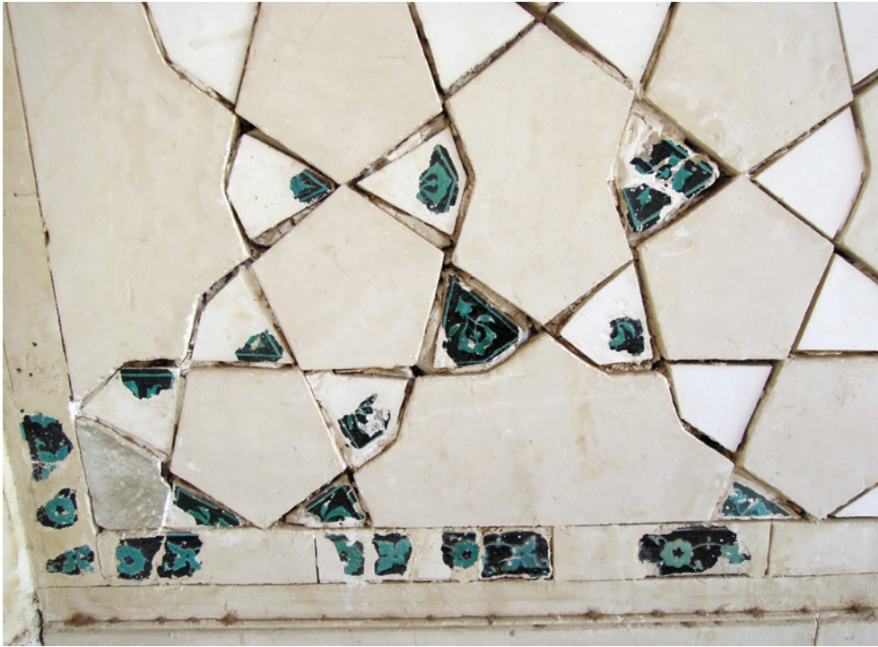
Fig. 18. Tabriz, Uzun Hasan Mosque, detail of a dado decoration displaying low-relief painted tiles with a black slip under a light blue transparent glaze. (Photo: Sandra Aube, 2014)
