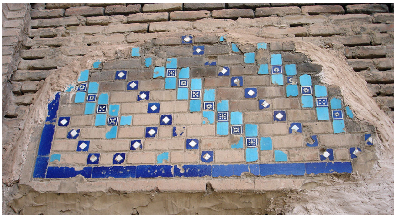
Fig. 5. Tabriz, Blue Mosque, blue-and-white square tiles mounted into a bannāʿī panel, (exterior walls of the mausoleum). (Photo: Sandra Aube, 2004)
