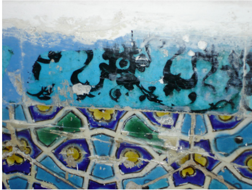
Fig. 20. Diyarbakır, interior of Safa Camii, detail of underglazed tiles painted in black under a turquoise glaze. (Photo: Sandra Aube, 2006)
