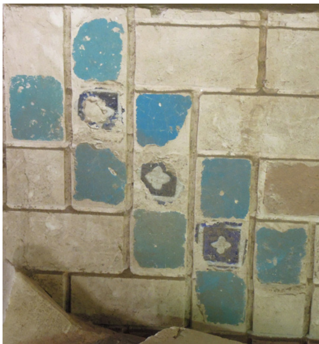
Fig. 4. Tabriz, Uzun Hasan Mosque, blue-and-white square tiles, restored into a brick panel (kept in the storeroom). (Photo: Sandra Aube, 2014)
