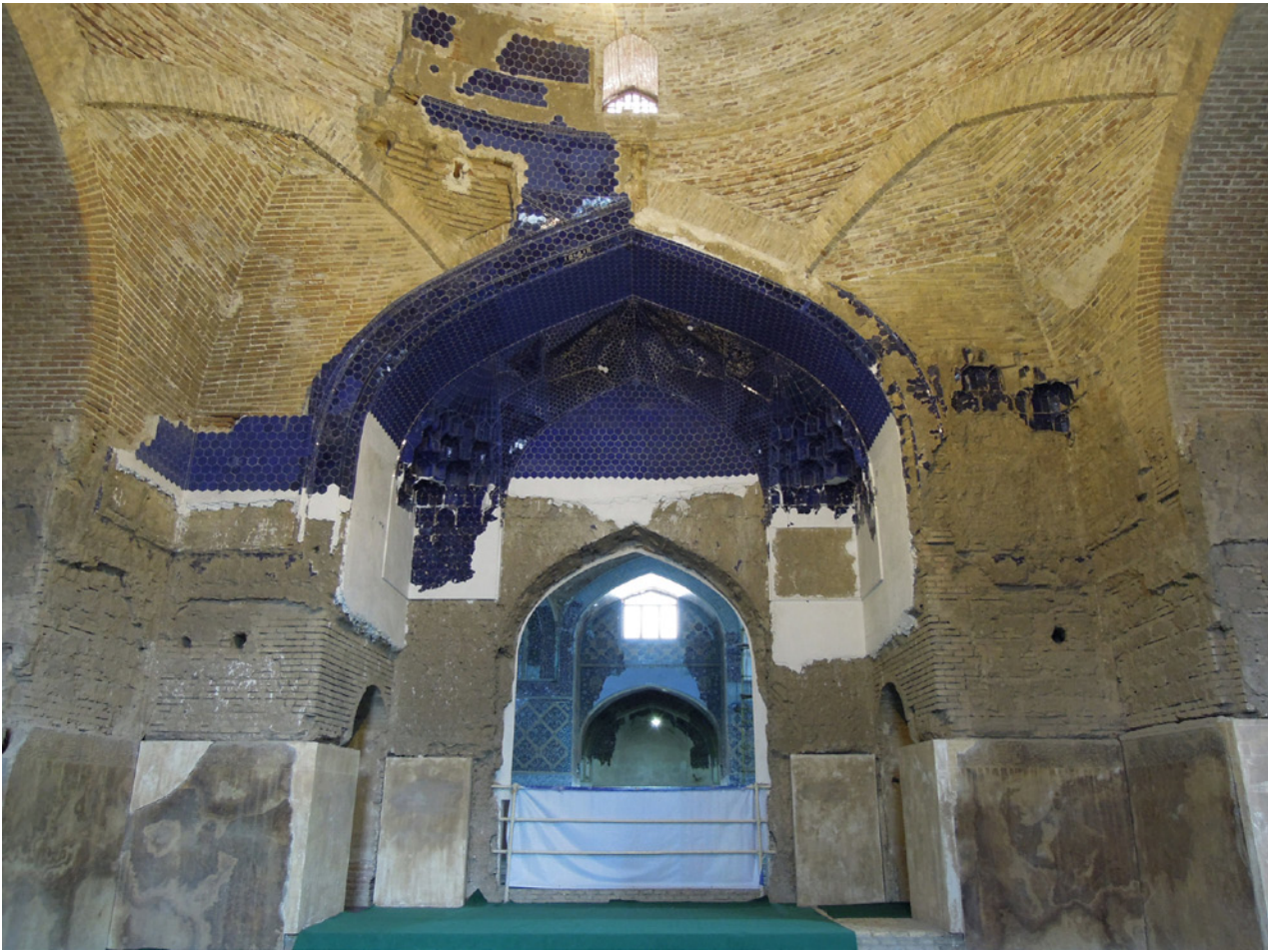
Fig. 23. Tabriz, Blue Mosque, cobalt and gilded tile decorations inside the mausoleum. (Photo: Sandra Aube, 2014)
