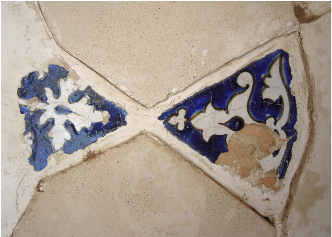
Fig. 17. Tabriz, Uzun Hasan Mosque, detail of two tiles from the dadoes of the qibla: on the right is an underglazed tile painted with cobalt and black on a white background (“blue-and-white” type); on the left is an overglazed tile painted with cobalt surrounded by a black line on a white glazed background (“black line” type). (Photo: Sandra Aube, 2014)
