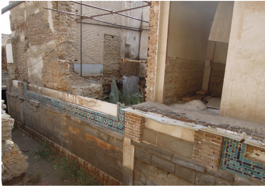
Fig. 3. Tabriz, Uzun Hasan Mosque, window frame with bannāʿī decoration. (Photo: Sandra Aube, 2014)
