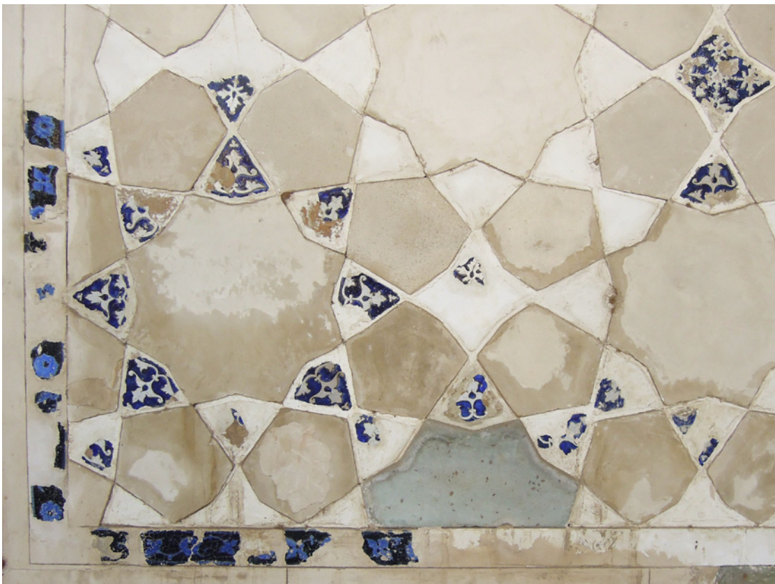
Fig. 16. Tabriz, Uzun Hasan Mosque, blue-and-white tiles in a geometrical network on the dadoes from the qibla side of the mosque. (Photo: Sandra Aube, 2014)
