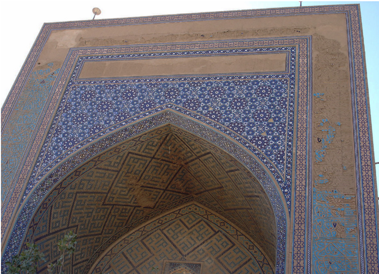
Fig. 34. Taybad, Zayn al-Din Mausoleum, detail of the spandrel decoration on the entrance iwan. (Photo: Sandra Aube, 2006)
