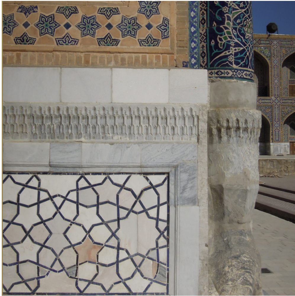
Fig. 37. Samarkand, Ulugh Beg Madrasa, fragment of dado decoration with marble column on projecting angles. (Photo: Sandra Aube, 2015)
