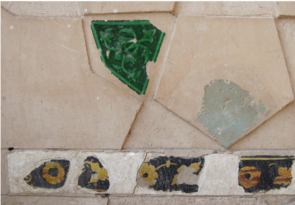
Fig. 19. Tabriz, Uzun Hasan Mosque, detail of a dado decoration featuring low-relief painted tiles with a black slip under a green or a yellow transparent glaze. (Photo: Sandra Aube, 2014)
