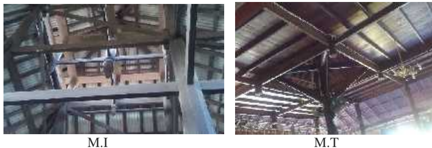
Figure 9. Roof structure of the two mosques (Photo by Laina)
