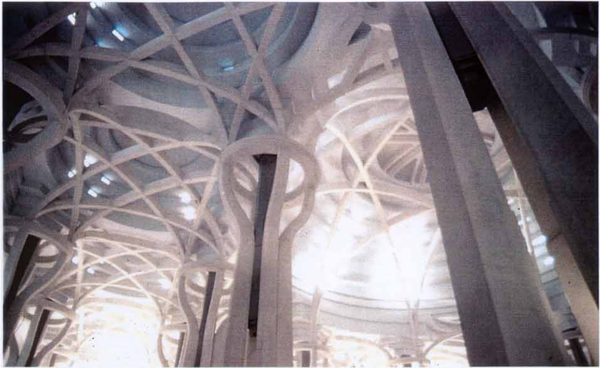
Above: The interior and exterior structural components throughout the complex also serve as decorative elements. In the prayer hall, four branches of the main concrete columns shoot out to form a web of arches and ribs that articulate the area beneath the domes.
