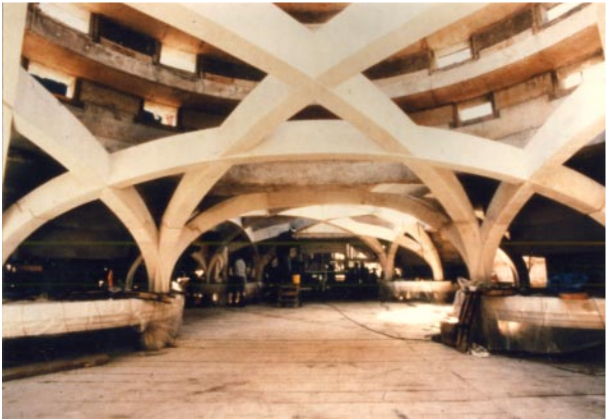
The Mosque during construction
