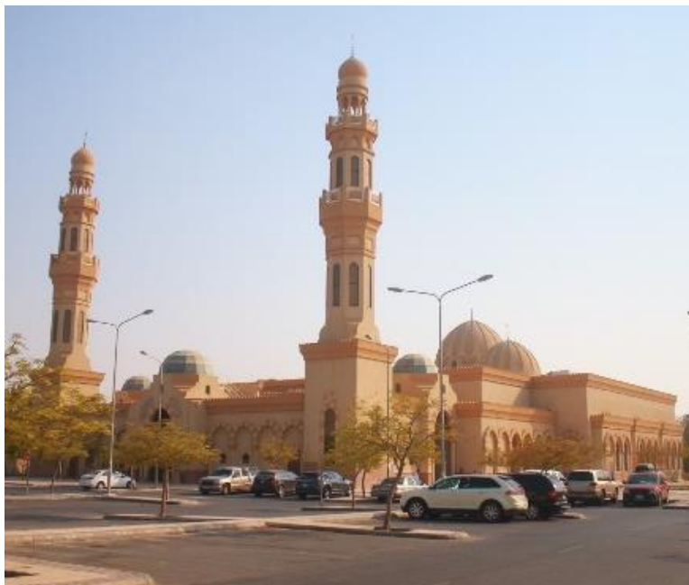
Figure 4.40. Parking, Farouq congregational mosque (Author, 2017).
