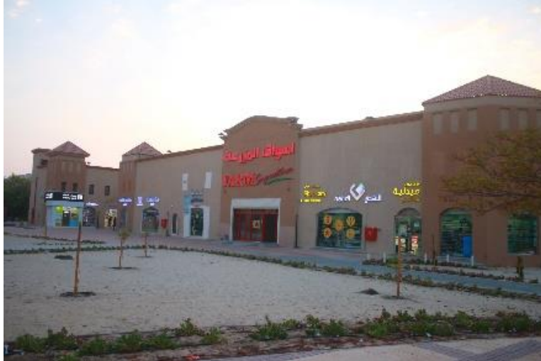
Figure 4.41. Adjacent services, Farouq congregational mosque (Author, 2017).
