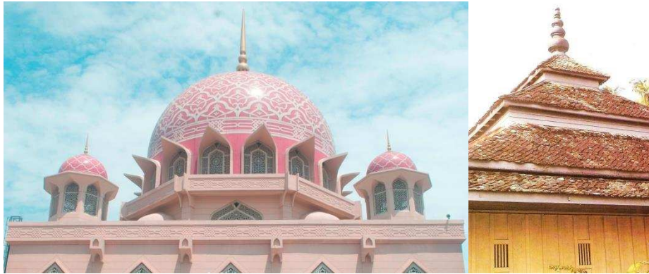
Figure 19: Comparisons between Putra Mosque (left) dome with influences of Middle East and (right) tiered roof of Kampung Tuan Mosque with buah butong.
