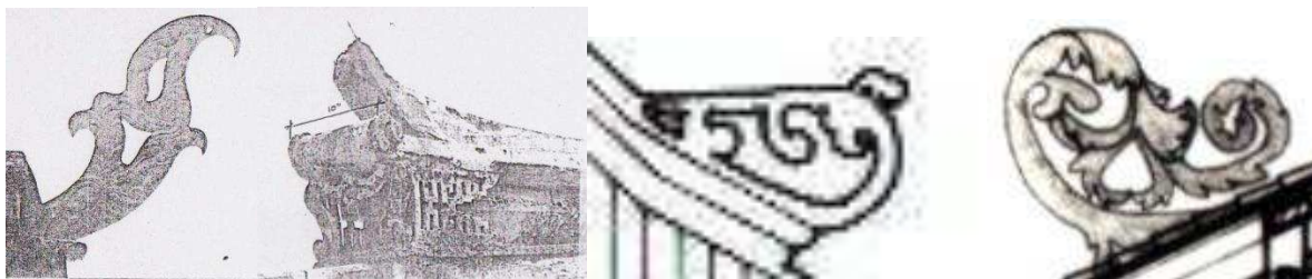
Figure 8: (left to right) Sulur bayung jenis figura and melentik respectively as used on Masjid Tengker Melaka ; jenis melingkar also called ekor itik (duck tails) used on Kampung Hulu Mosque, Melaka; jenis melingkar (ekor itik) used on a Langgar Mosque, Kelantan.
