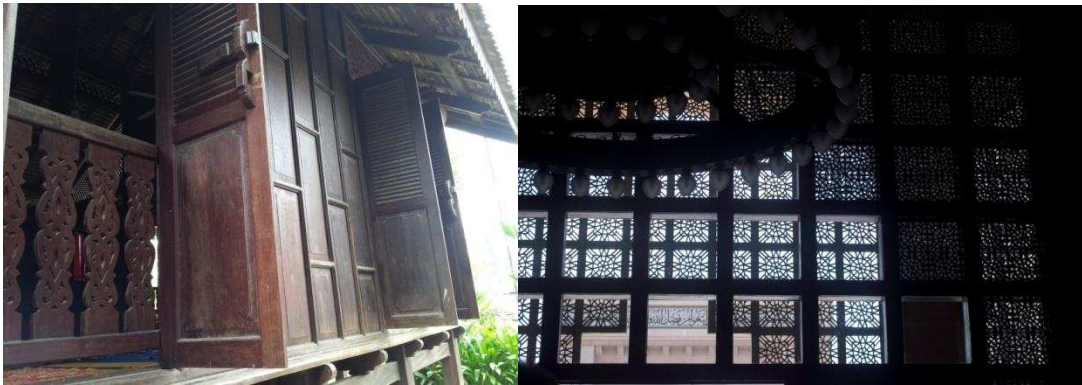
Figure 23: Shows an opening and natural ventilated prayer space by using ornamentation at Seberang Jerneh Mosque (left) and enclosed ornamentation of Middle East at prayer hall in Putra Mosque (right).
