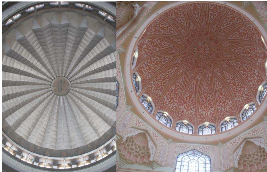
Figure 20: Comparison of Sultan Mizan Mosque interior dome ornament (left) and Putra Mosque (right) to differentiate between imitation Middle Eastern elements and the use of modern concepts.
