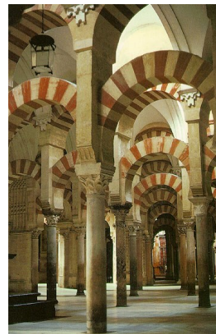
Figure 5: Two levels of horseshoe arches with alternate color blocks inside La Mezquita - the Great Mosque of Cordoba.
