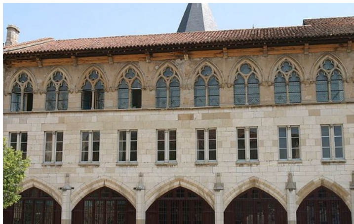
Figure 10: Rebuilt façade of the Church of Cluny
