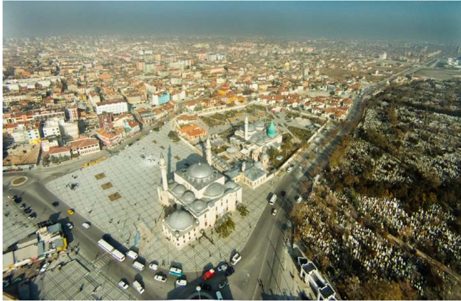
Figure 8.b Aslanlıkişla road, which separates Mevlana Museum from the Üçler Cemetery and thus causes a faulty ontological arrangement
