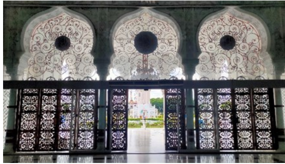
Figure 5. The overall look of the door in MRB [source: Author]
