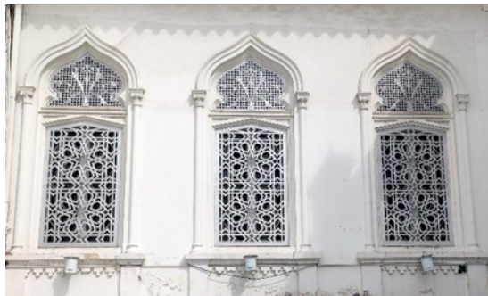
Figure 6. The window in MRB [source: Author]
