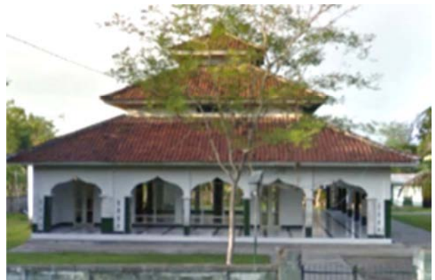
Figure 26. Al Mujahidin Mosque, Simbar sub-village, Bayan village, with a model of stacking roof 3 of tile.
