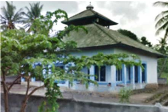
Figure 29. Nurul Iman Mosque, Obel-Obel village kec. Sambelia, tile roofs stacked in two.
