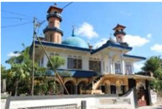
Figure 62. Exterior of the Nurul Hidayah mosque in Batutulis village Jonggat sub-district, central Lombok district.
