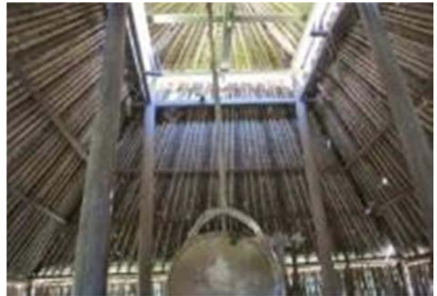
Figure 25. Ancient Mosque interior in the village of Bayan, North Lombok Regency.
