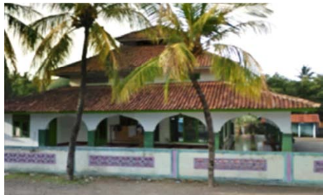
Figure 27. Nurul Hidayah Mosque Belanting village Bayan sub-district, also with a three-tiered roof model.
