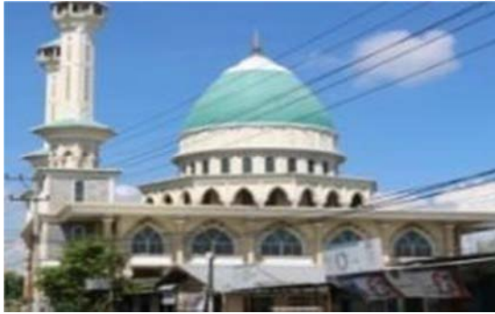
Figure 36. The tebolak dome in Darul Hidayah Mosque in Cermen hamlet, sub-district Cakranegara.
