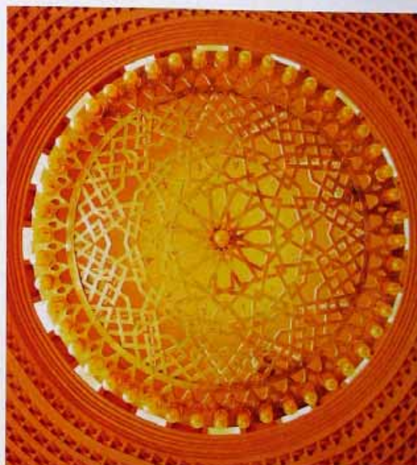
(Above) A view into the main dome of the Al-Harithy Mosque (1986), Jeddah (see p. 39), one of the series of mosques designed by Abdel Wahed El-Wakil, showing the intricate brick construction of the pendentives and the geometric pattern of the chandelier.
