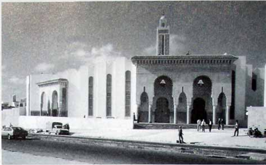
(Above) The street façade of the King Abdul Aziz Mosque and Foundation, Casablanca, by Coteba International. Completed in 1983 and dressed in acceptable ornamental garb, the mosque was built and decorated in the space of ten months using many prefabricated elements.
