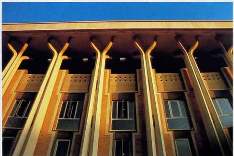
(Right and opposite) Exterior details showing the library with its floating slab roof supported by externally expressed columns, and the freestanding minaret, 40 m (130 ft) in height, with two-tiered galleries.
