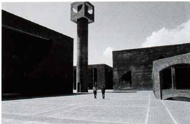
(Above) The ceremonial entrance portal, set at one corner of the site and consisting of five freestanding arches, gives access to the Islamic Centre for Technical and Vocational Training and Research (1978–87), Dhaka. The design for the entire complex by the Turkish firm Studio 14 was guided by the principles of the historic Ottoman külliye layout. The freestanding minaret marks the centre of the complex and also serves as a rotational pivot for pedestrian circulation around the mosque.
