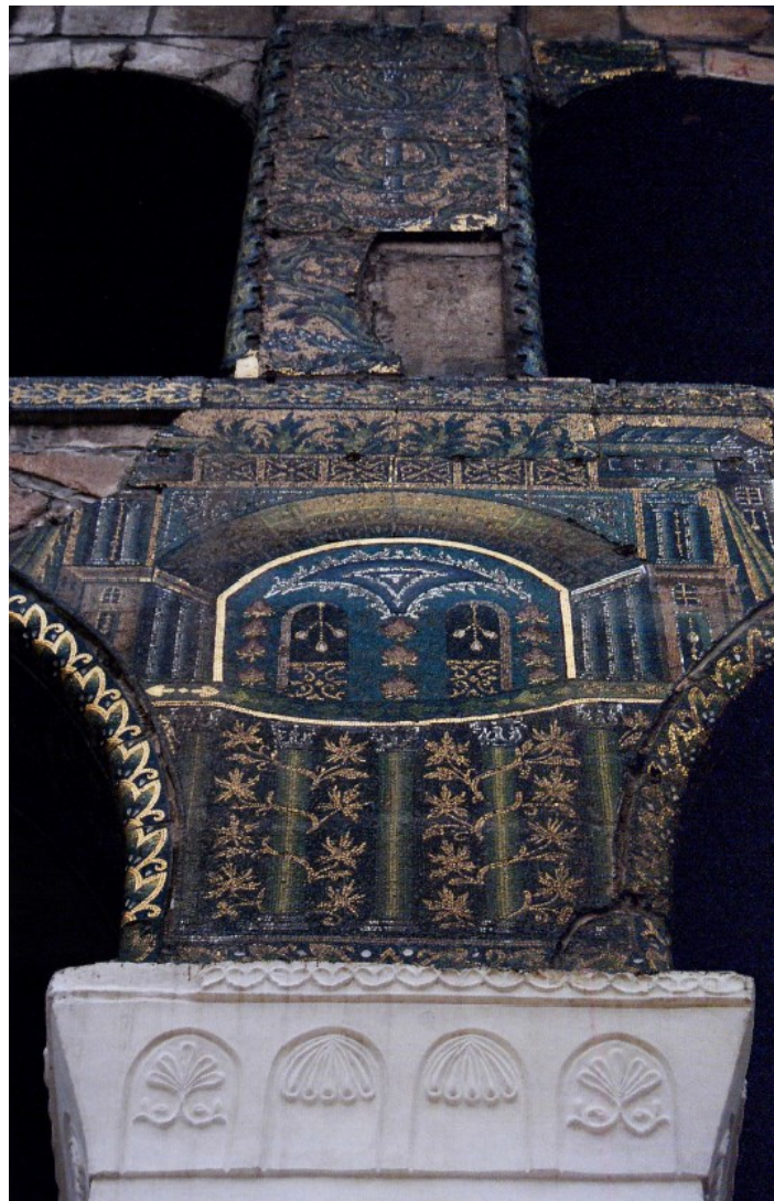
West courtyard pier with mosaics set in modern concrete
