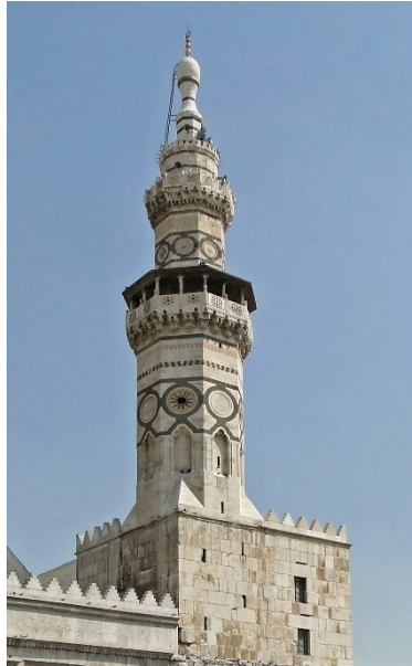
Minaret of Qaitbay, constructed in 1488 on the orders of Sultan Qaitbay Source: Bernard Gagnon
