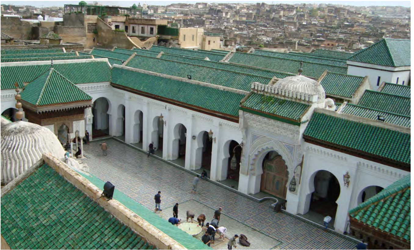
Renovated courtyard viewed from the roof.
