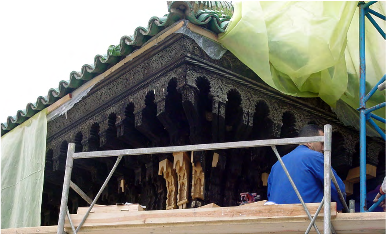
Resoration of the entrance wooden canopy.
