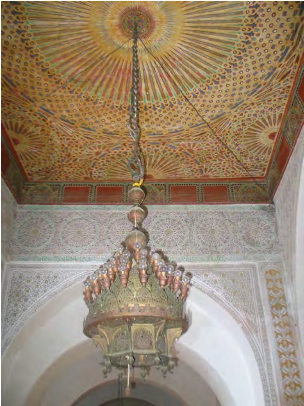
Wood ceiling and lamp, before and after restoration.
