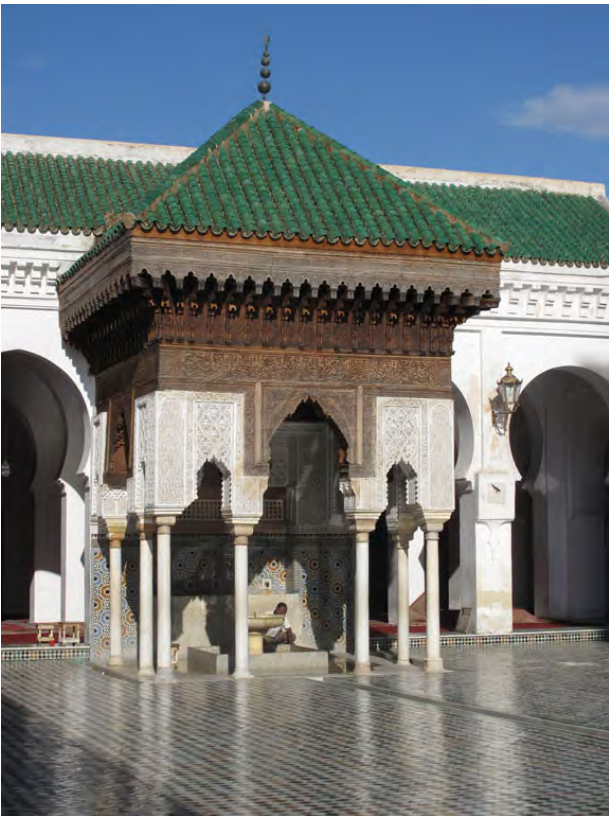
Details of the restored fountain in the courtyard.
