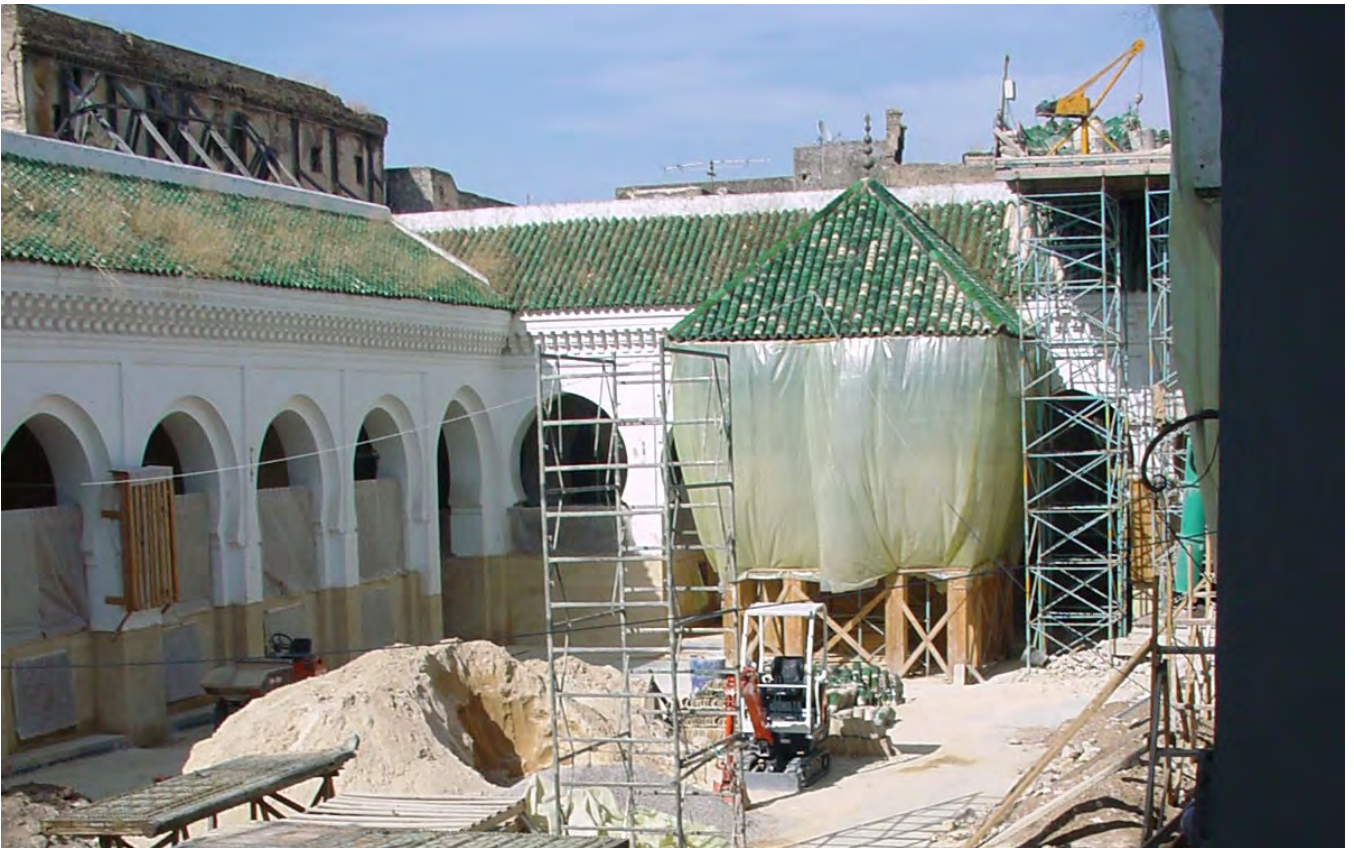
Restoration work in the courtyard.
