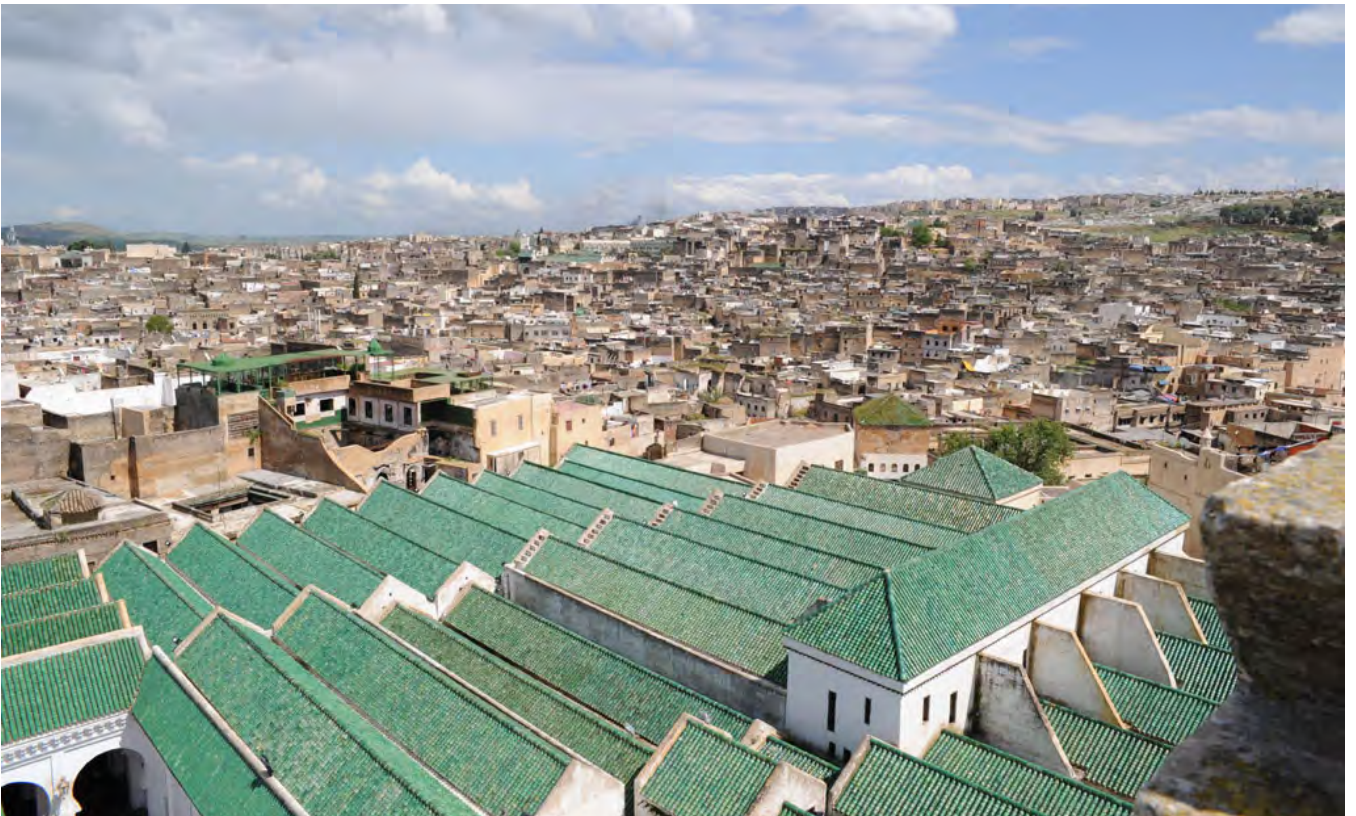
View of the roof restored.
