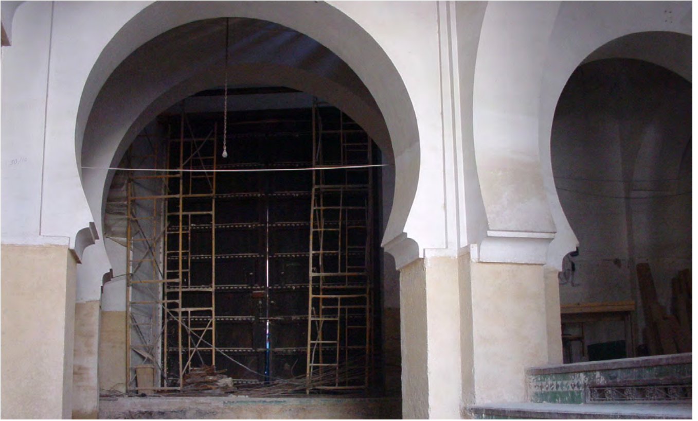
Restoration work in the prayer hall.
