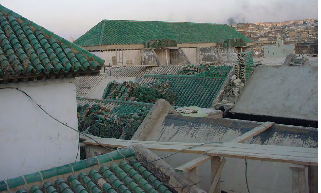
Restoration of tiles on the roof.
