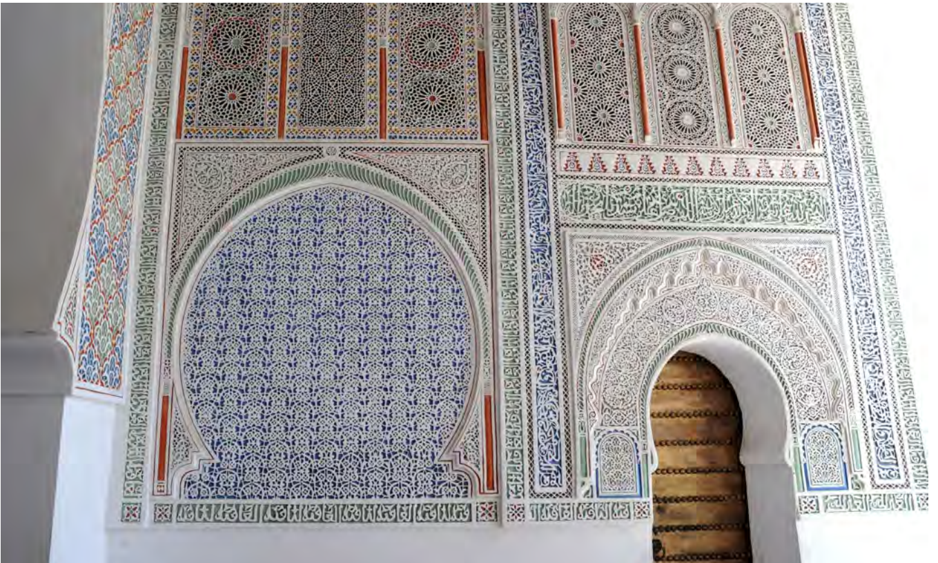
Stuccos after restoration.
