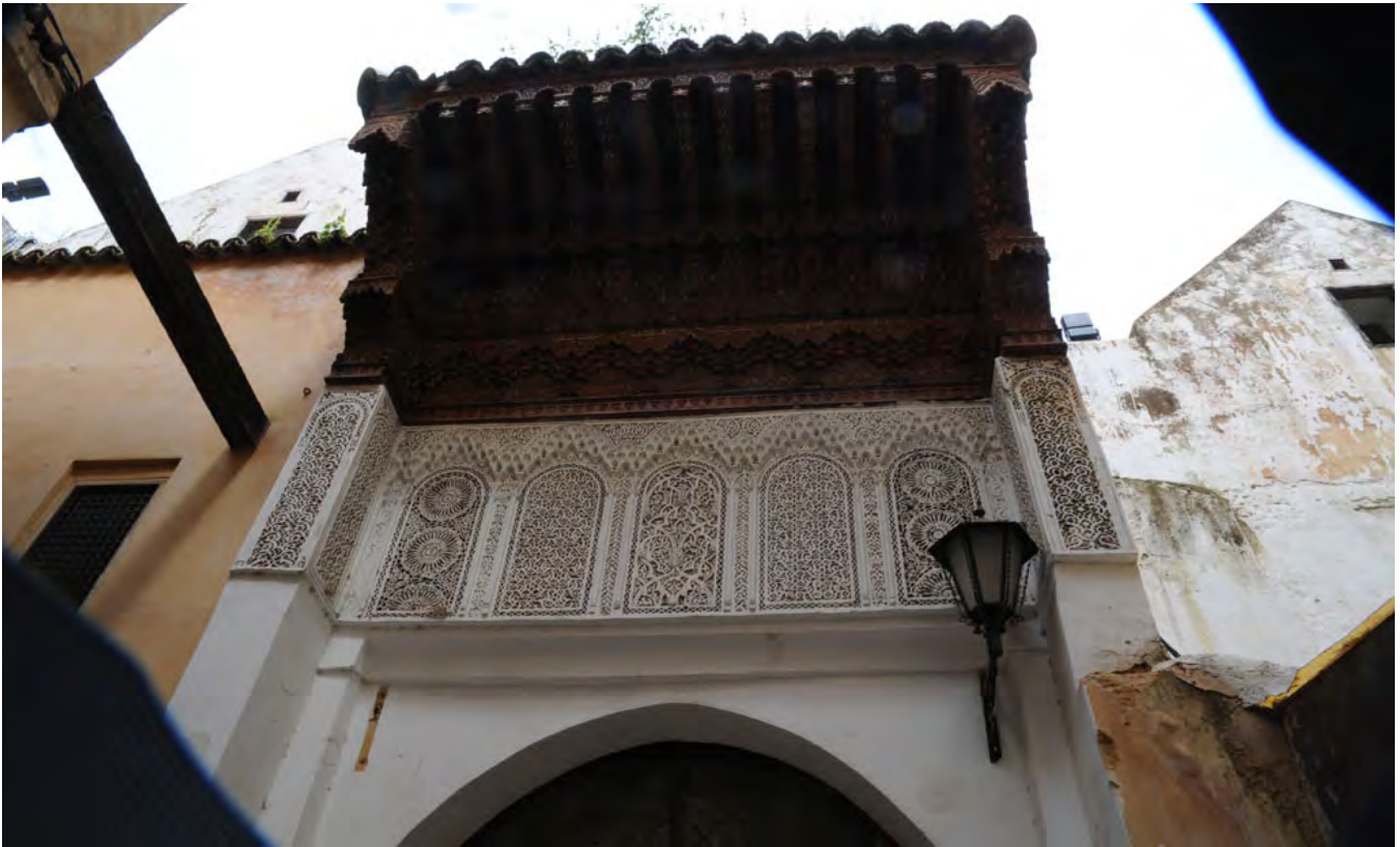
Restored wooden canopy.
