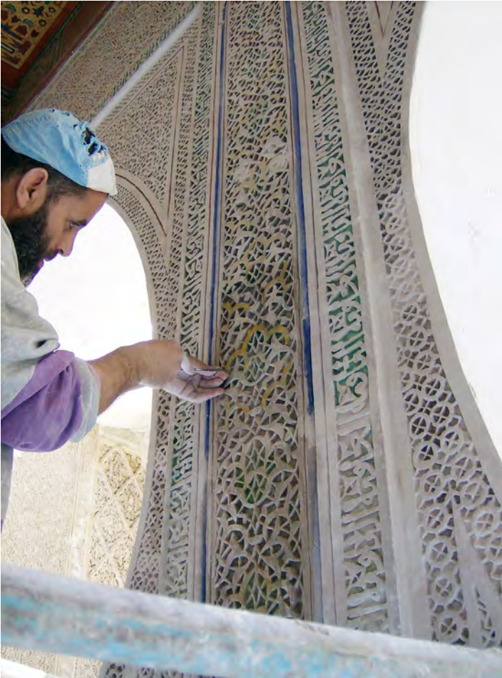
Restoration of stuccos.
