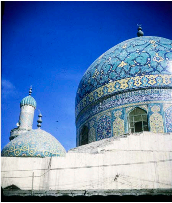
Figure 20. Glazed tiles used as veneer over a brick core, like those used in this Baghdad mosque, were common in the Islamic world from ‘Abbāsīd times onward. Their use reached its zenith in Iran and Turkey during the sixteenth and seventeenth centuries. (Photo by Ronald B. Lewcock)
