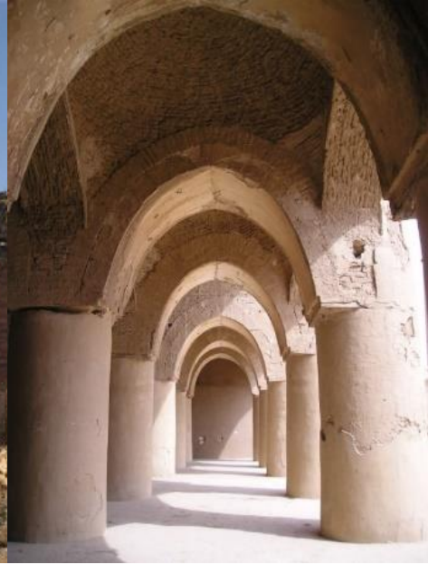
Figure 248: Tarik Khana Vaults , 750-789 AD
