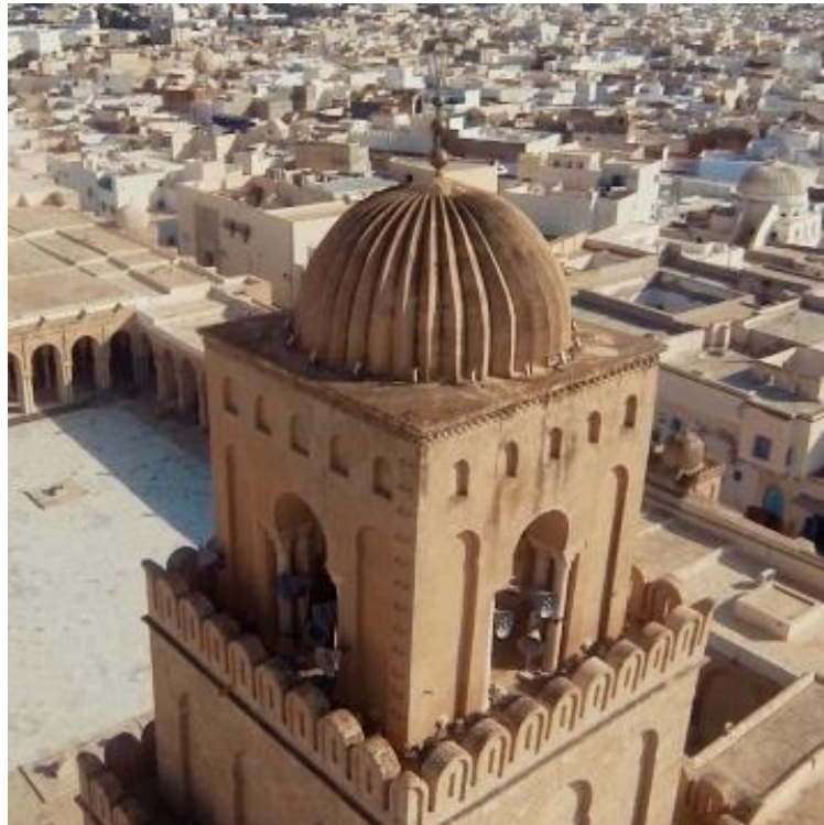
Figure 9: Minaret Dome Exterior View.
