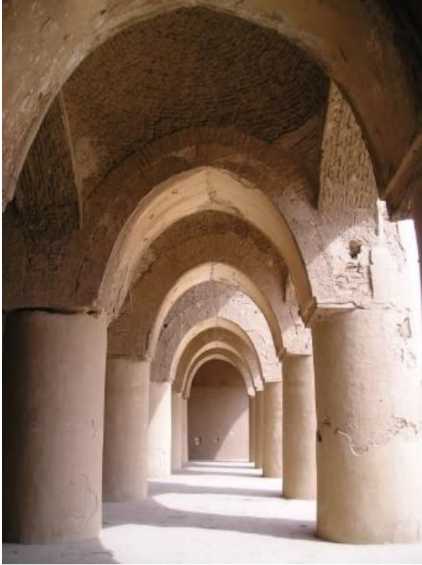
Figure 231: Pitched-brick Vaulting in Tarik Khana
