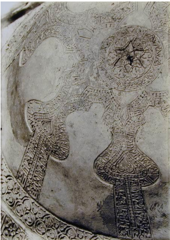
Figure 200: Stucco of Al Mihab Dome
