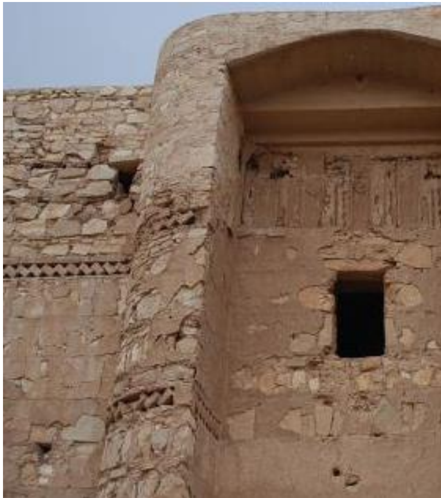
Figure 54: Qasr Harranah Entrance Brick Method, 710 AD Source: Guide
