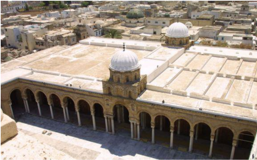
Figure 12: Zaytuna Court with Chamber Hall View.
