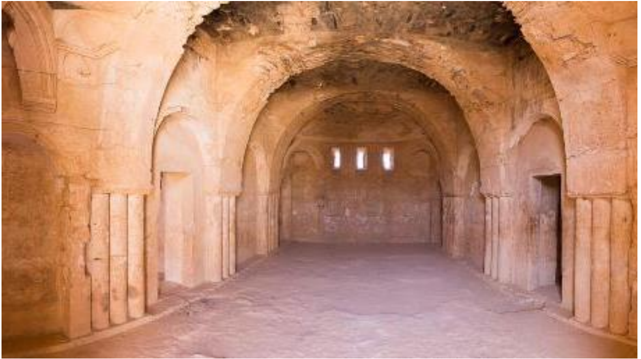
Figure 55: Barrel Vaults, Qasr Harranah Source: Trip Advisor
