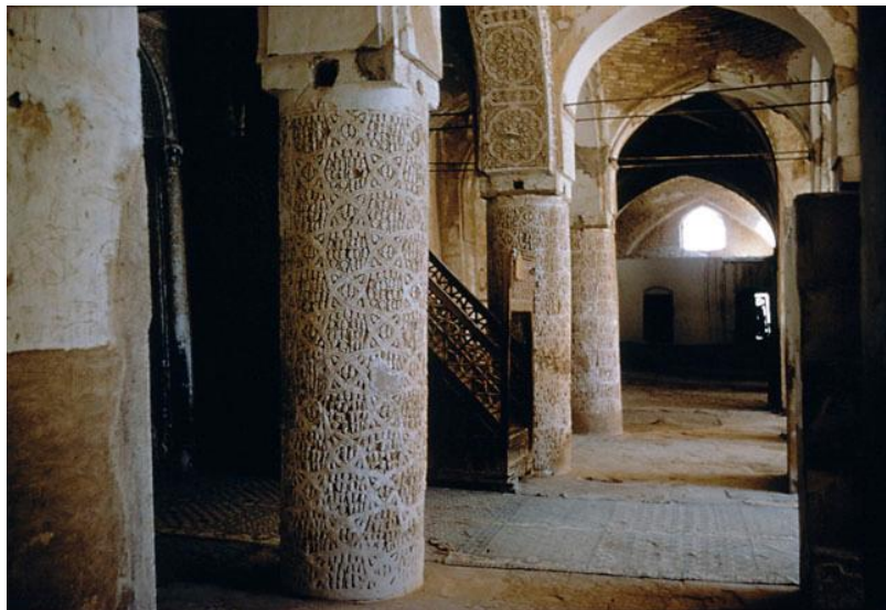
Figure 237: Na'in Pitched Brick Vaults
