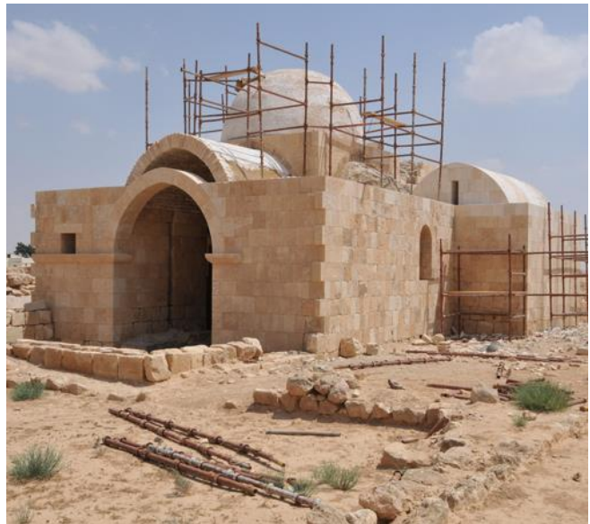
Figure 81: Hammam Al Sarah, after restoration
