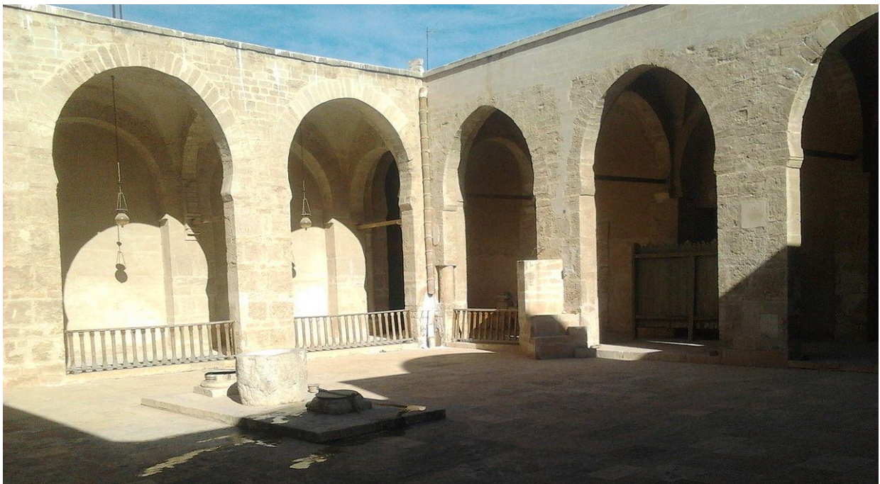
Figure 218: Sfax Chamber corridor vaults
