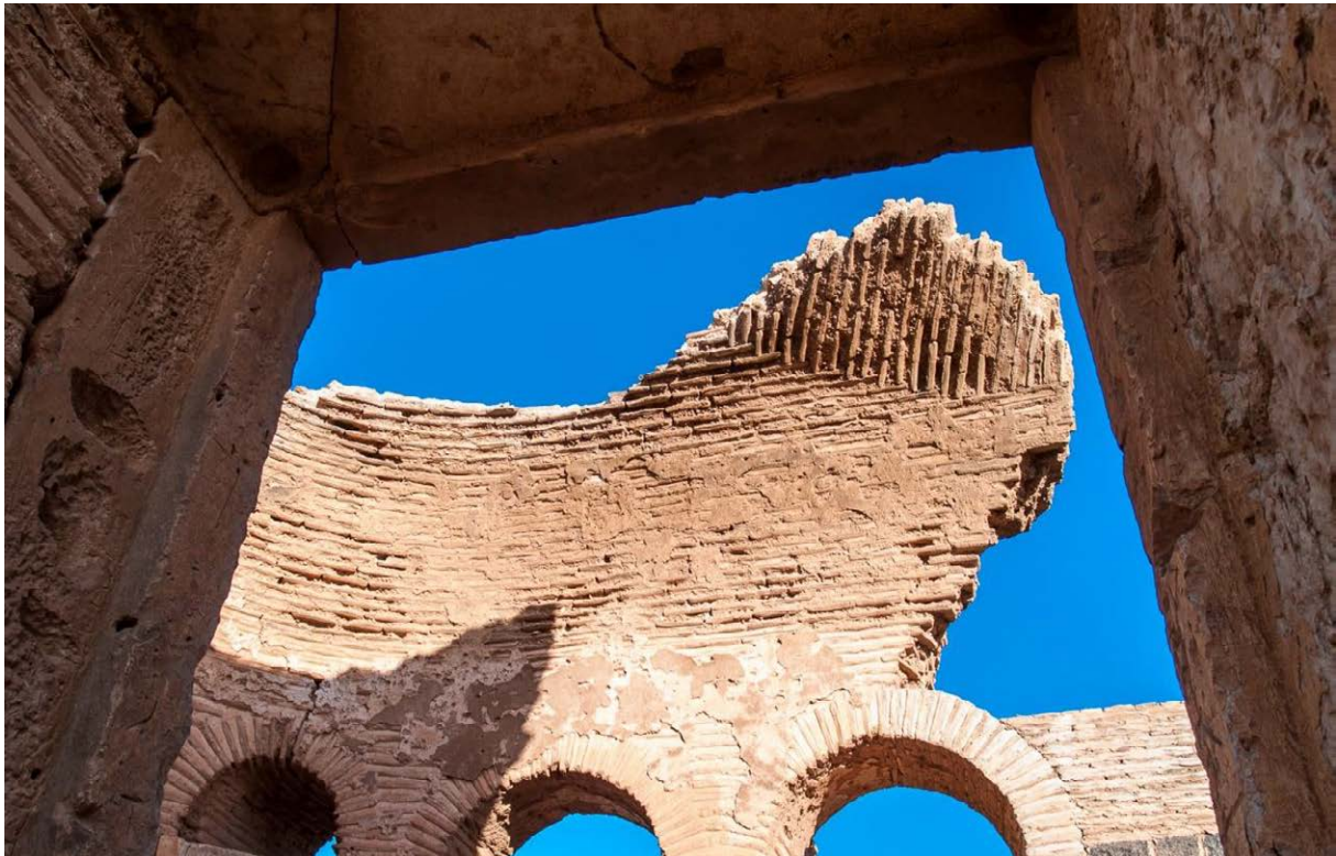
Figure 45: Qasr Ibn Wardan Mixed Brick and Stone Masonry of Byzantine Tradition
