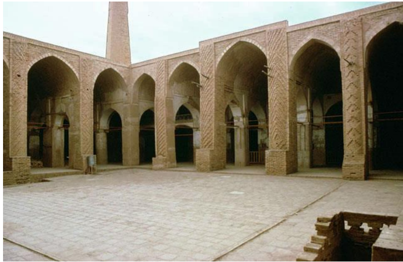
Figure 236: Na'in Pitched Brick Vaults.
