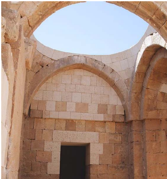
Figure 80: Hammam Al Sarah while restoration
