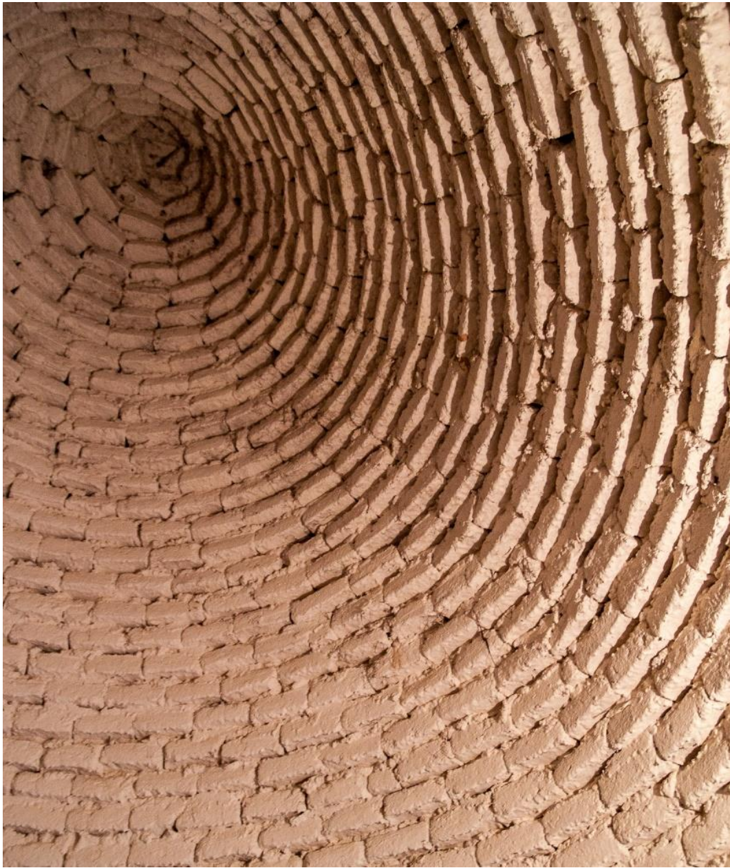
Figure 180: Brick Method in Libya, Atique Mosque
