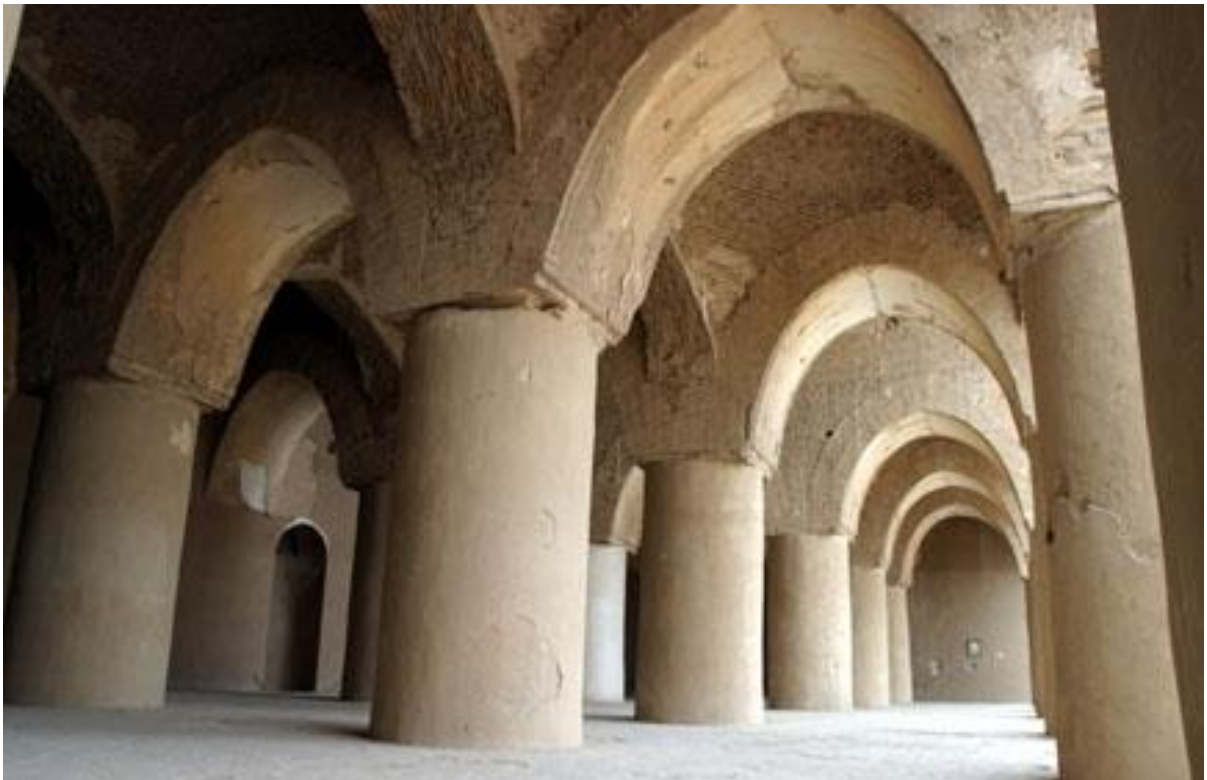
Figure 233: Pitched-brick Vaulting in Tarik Khana, 750-789AD
